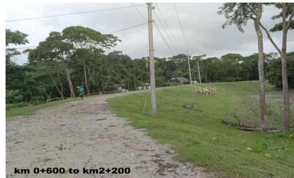
Figure 3-30: Embankment Turfing work at km 0.600 in Polder-43/2C
