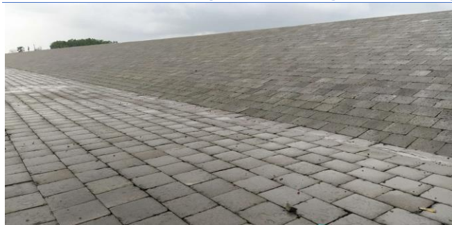
Figure 3-13: Nalian Closure Dam of Polder-32
