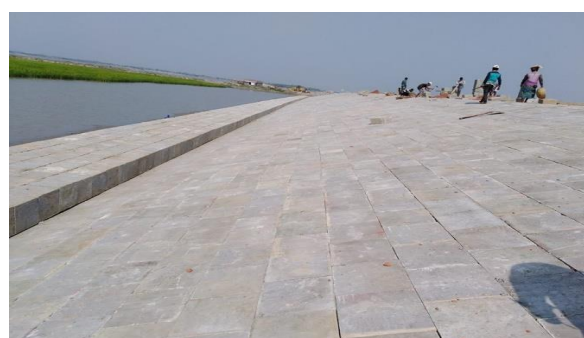
Figure 3-10: Completed Slope Protection Works in Polder-32
