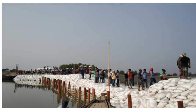
Figure 3-11: Nalian Closure Dam of Polder-32 (completed)
