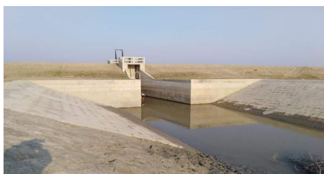
Figure 3-9: Completed DS of Polder-32
