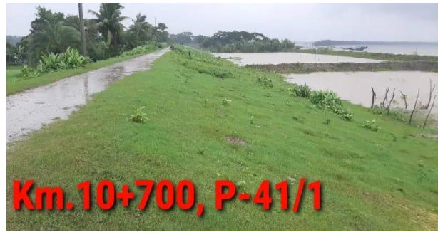
Figure 3-28: Embankment Turfing work at km 10+700 in Polder-41/1
