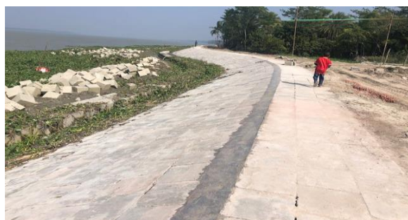
Figure 3-25: Bank Protection with Pitching Works (Polder 39/2C)
