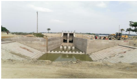
Figure 3-27: Ongoing DS-3 In Polder-43/2C
