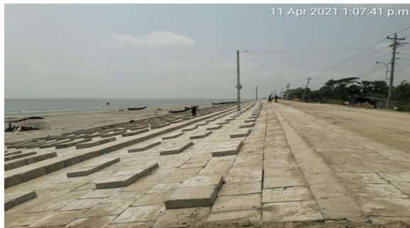
Figure 3-29: Slope Protection work For KM 30+800 to Km 31+450 in Polder-48
