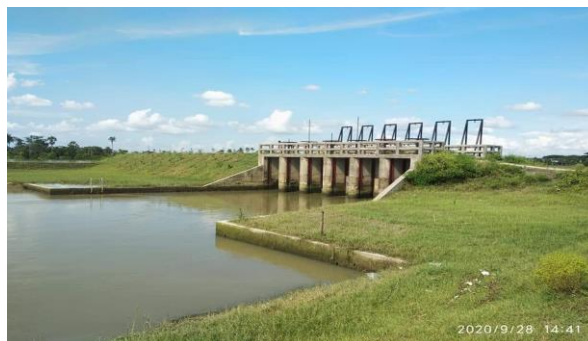
Figure 3-16: DS-6 of Polder-35/3 (Completed)
