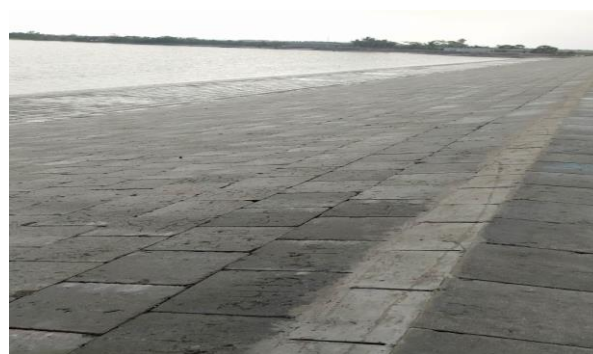
Figure 3-12: Nalian Closure Dam of Polder-32 (completed)
