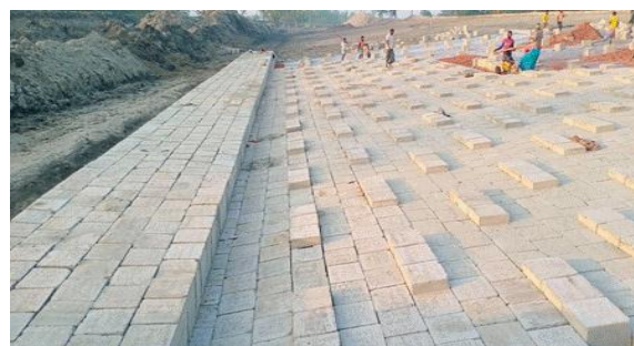
Figure 3-26: Ongoing Slope Protection Works (Polder 40/2), Barguna
