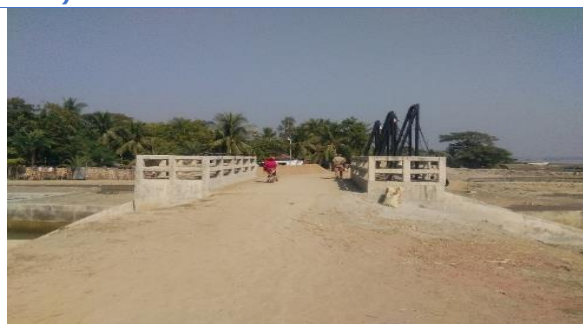
Figure 3-14: Completed DS-10 of Polder-33
