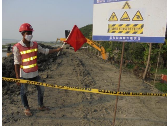
Image-10:Engagement of Signal man during embankment construction works in P-39/2C, Package-2
