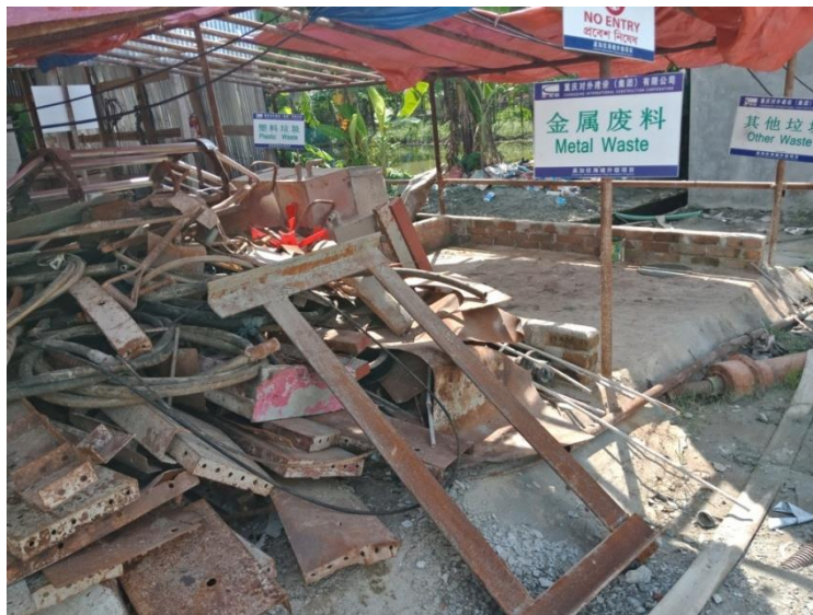
Image-12: Proper storing of industrial wastes in P-41/1, Package-2
