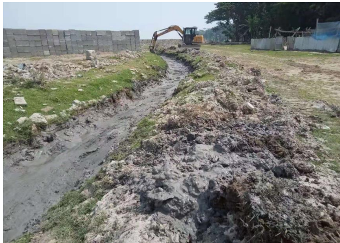
Image-8: Improving drainage system for avoiding water logging in P-39/2C, Package-2
