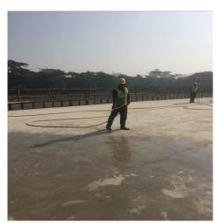
Worker sprinkling water in worksite to control dust
