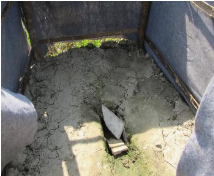
Opened latrine used by the workers
