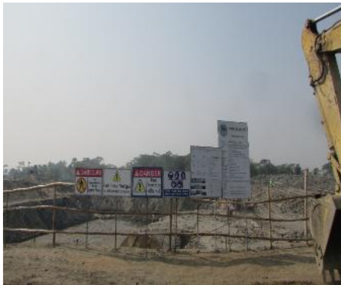
Erection of safety and cautionary signboard, signage and symbols
