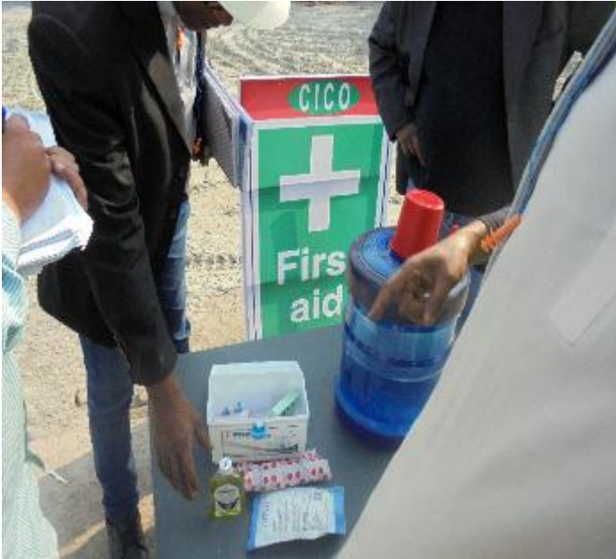
First aid box in work site
