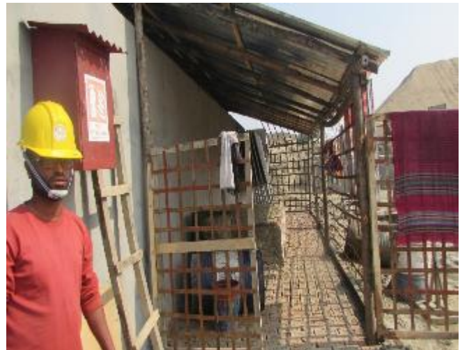
Fire extinguisher in box for protection from sun and rain
