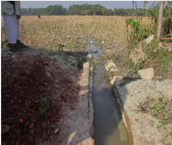
Drain from CC block manufacturing yard directly opened to agriculture land
