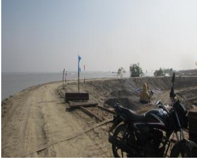
Pedestrian alternative passage way with DS work site
