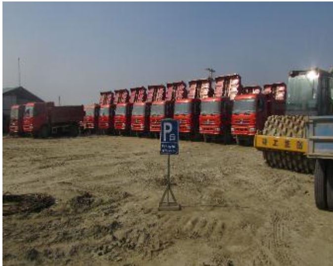
Designated parking are with signage
