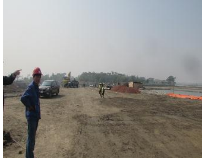
Sprinkling of water to control dust
