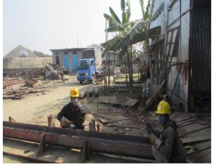
Welding workers using PPE
