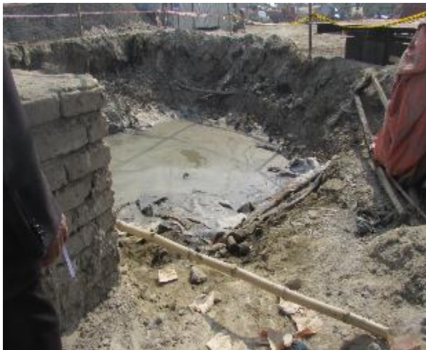
Decanting ditch with the discharge of the CC block manufacturing plant
