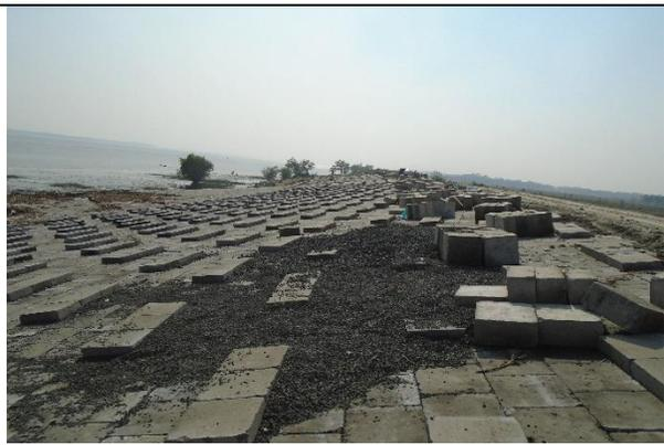
Bank Protection work has been completed but crushed stones are around later in the Ch: km 16+774 under polder-35/1.
