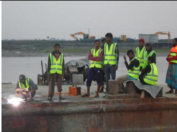
Workers welding work without using proper PPE at Nalian Closure Dam under polder-32
