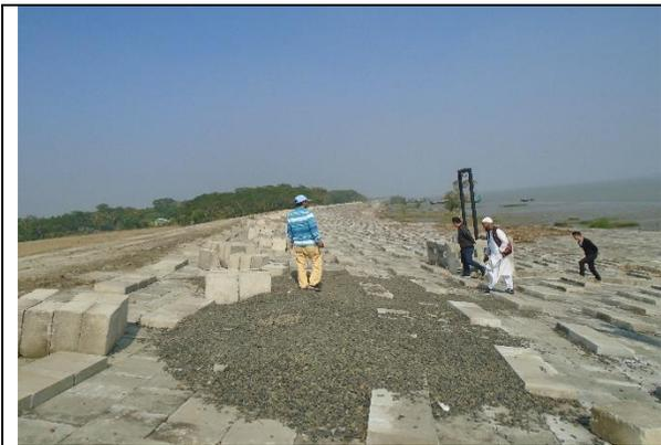
Structure work has been completed but gate not yet installed, and crushed stones are around FS-5 under polder-35/1.
