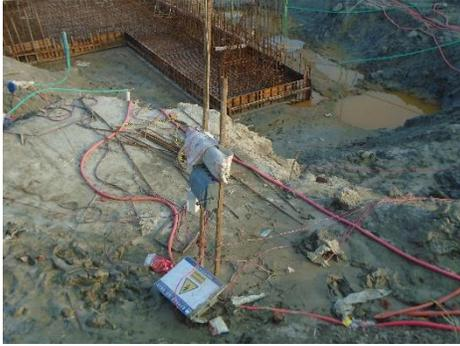
Electric wire haphazardly on the ground at DS-2/A under polder-48
