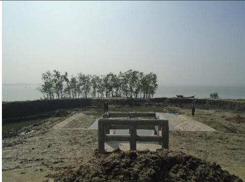
Structure work has been completed but gate not yet installed, and water logging for a long time at DS-8 under polder-41/1.
