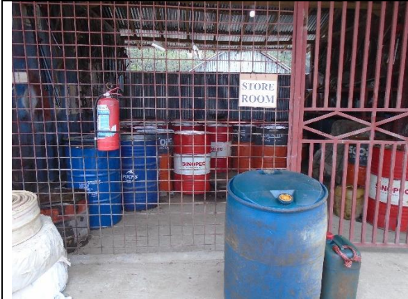
Separate storeroom for oil & lubricant at Nadmullah CC Block manufacturing yard under polder-39/2C
