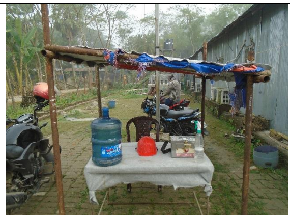
Supply of drinking water and First Aid box for the workers at Burirchar CC Block manufacturing yard under polder-41/1
