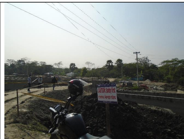
Presence of demarcation at DS-1 under polder-43/2C
