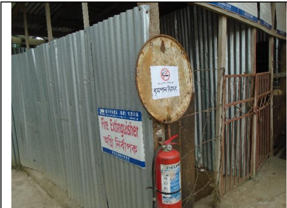
Fire extinguisher with expiry date presence on the work site at Nadmullah CC Block manufacturing yard under polder-39/2C
