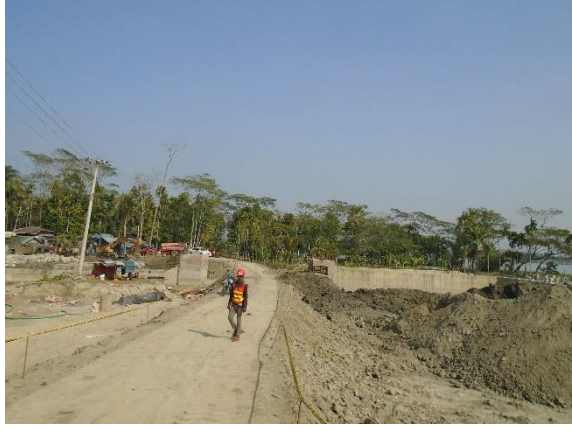
Presence of demarcation at DS-1 under polder-43/2C
