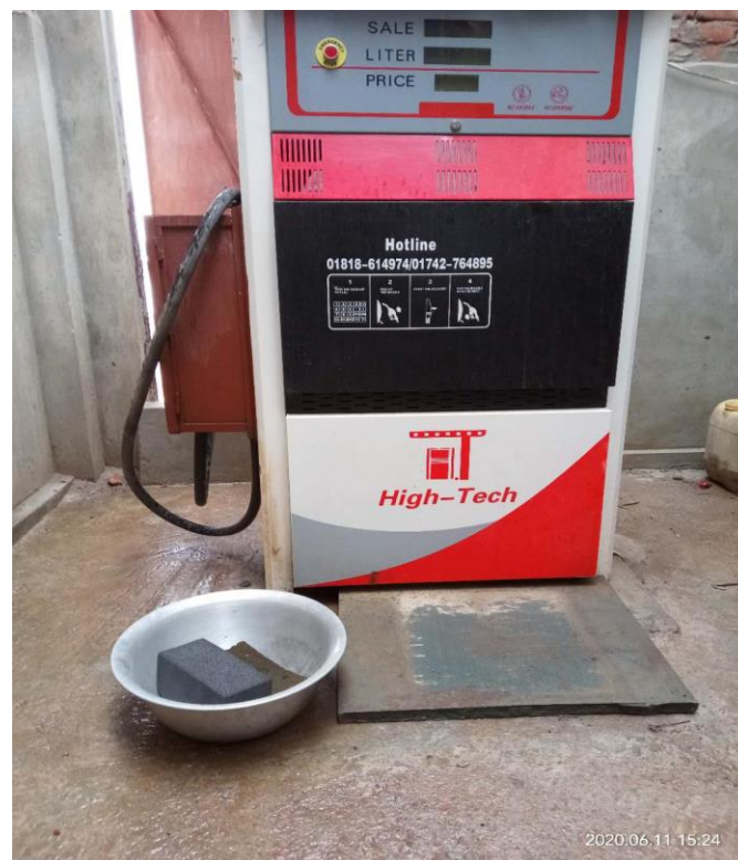
Fig. 14: Absorbent mats to manage oil leakage at P-39/2C, Package-2
