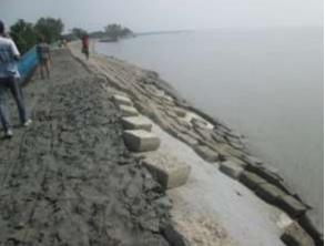
Photograph 5.2: Deteriorated Condition of Existing Slope Protection Work
