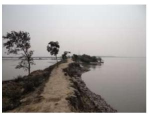
Photograph 6.4: Vulnerable condition of embankment near Golkhali
