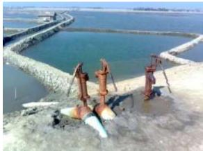
Photograph 6.6: Hand tube-wells on the embankment caused damages
