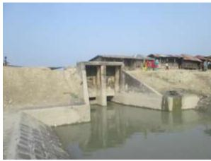
Photograph 5.3: Fully damaged condition Photograph of Rw DS-1 (Padmapukur) condition of
