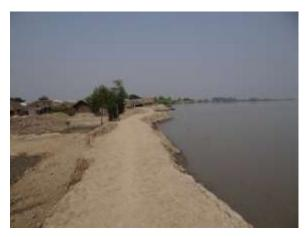
Photograph 6.5: Vulnerable condition of embankment along Sakbaria river
