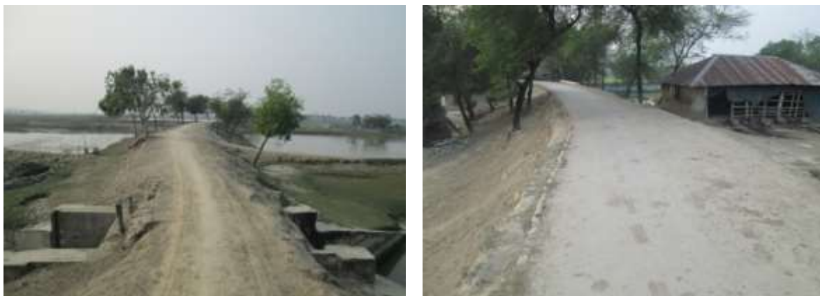
Photo 5.1: Present condition of the embankment of the Polder
