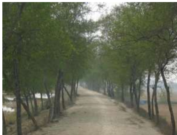
Photo 6.25: Bablatreesplanted along the embankment
