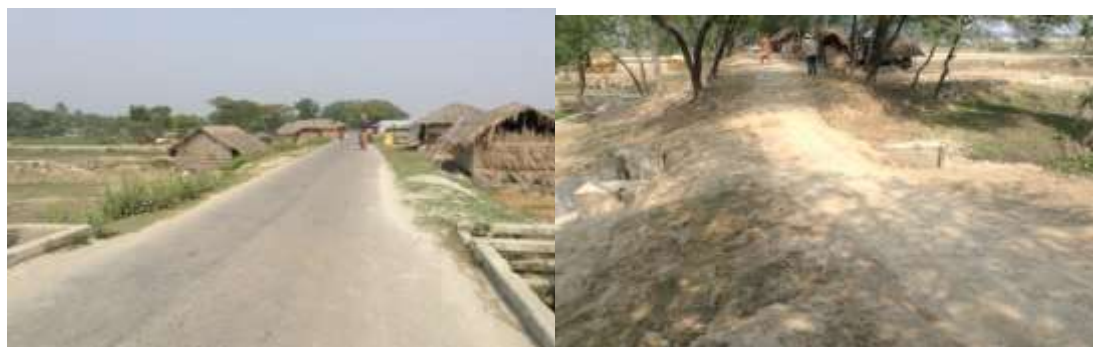
Photo 5-3: (a) WAPDA road on the embankment (b) Deplorable condition of the embankment (D/S-5)
