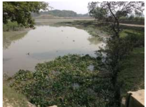
Photo 5-2: Narrow drainage khal (D/S-5) due to siltation and vegetation
