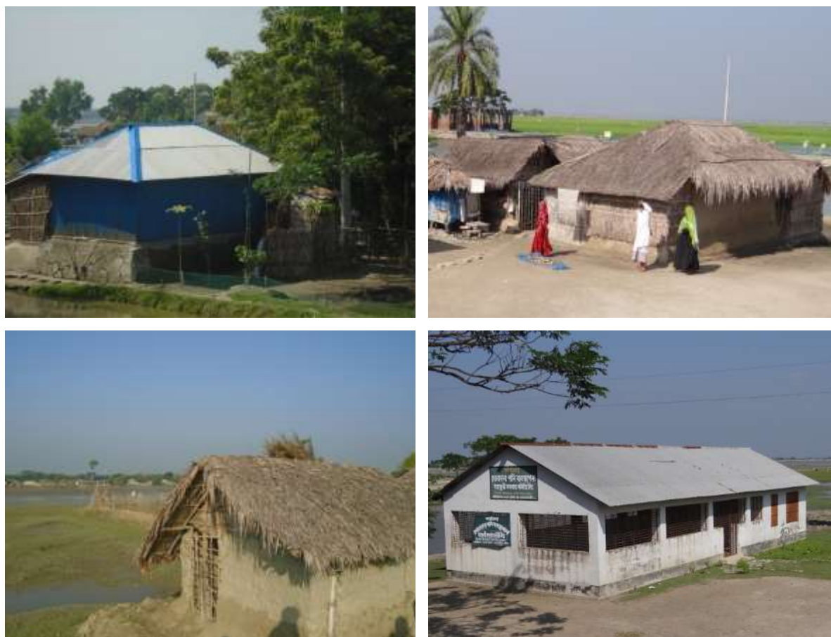
Photograph 6.26: Different types housing structure at the Polder area
