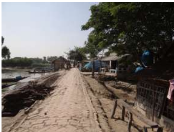
Photo 5-2: Brick soling on the crest of the embankment
