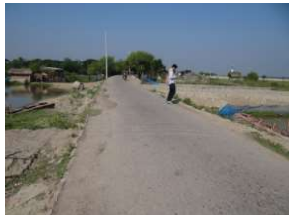
Photo 5-3: Bitumen carpeting on the crest of the embankment
