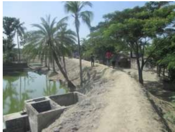
Photograph 6.6: Vulnerable condition of the embankment at Paschim Kanmukhi
