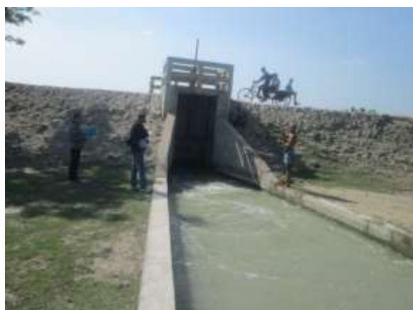
Photo 5-5: Functioning condition of DS-1
