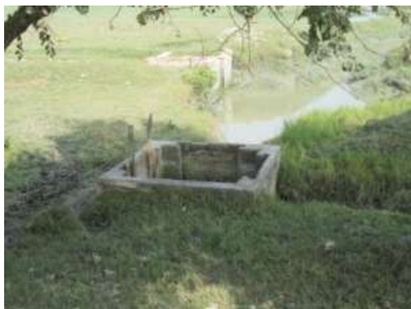
Photograph 5.4 : Flushing sluice over Amtoli khal
