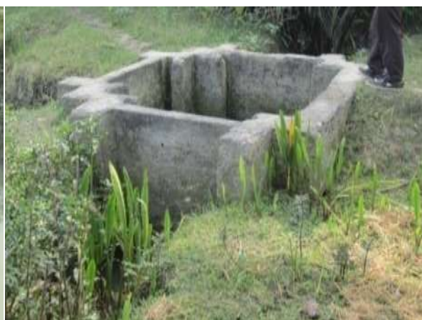
Photograph 5.7 : Flushing sluice at Lashmi khali
