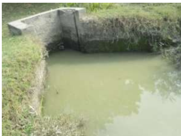
Photograph 5.6 : Flushing sluice at Purba sayra
