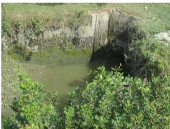
Photograph 5.3 : Flushing sluice at Gomoti
