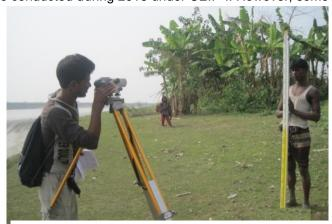
Figure: Embankment Cross section Survey
