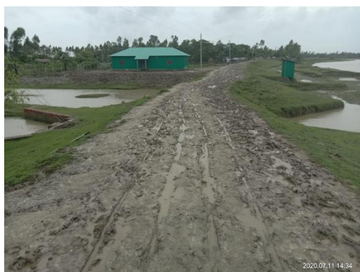
Figure. Sluice-10 of P-64/1A
