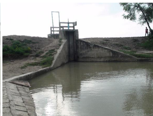
Figure: Asanghar Sluice of P-29
