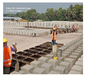
Figure 3-56: Casting the CC block in the camp of Polder-40/2
