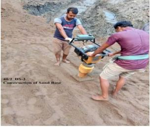
Figure 3-57: Construction of the sand base of DS-02 of Polder-40/2
