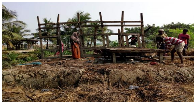
Figure 3-15: House relocation at FS-1 in Polder 35/3
