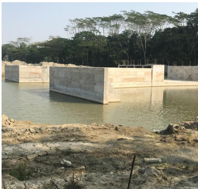
Figure 3-55: Site View of Completed Sluice—DS-12 of Polder 39/2C
