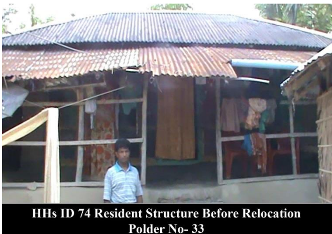
Figure 3-7: HH 74 Before relocation of Polder-33
