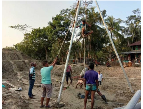
Figure 3-58: Dewatering for FS -9 of Polder 40/2
