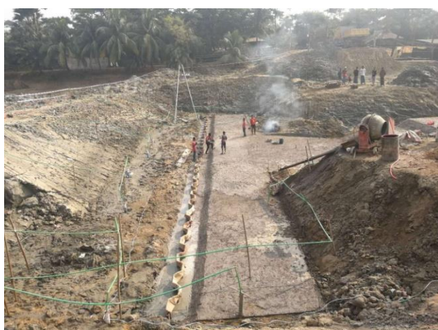
Figure 3-63: Dewatering for DS-3 of Polder 47/2
