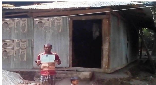
HHs ID 1732 Resident Structure After Relocation Polder No. 35/1
