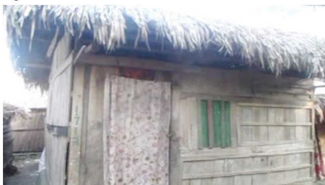
HHs ID 1713 Resident Structure Before Relocation Polder No. 35/1
