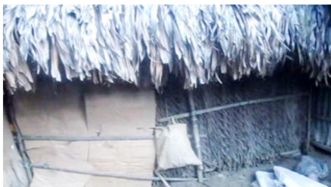
HHs ID 1712 Resident Structure Before Relocation Polder No. 35/1
