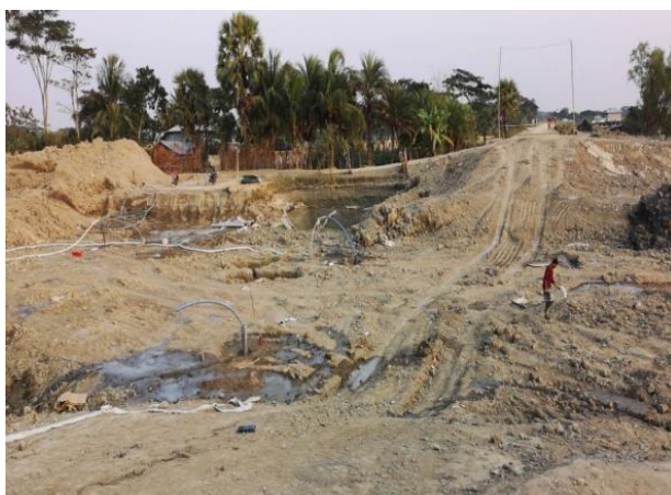
Figure 3-63: Dewatering for DS-3 of Polder 47/2
