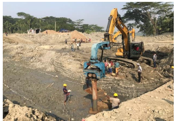
Figure 3-60: Executing the sand pile for DS-8 of Polder-41/1
