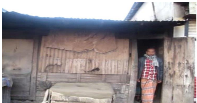
HHs ID 1732 Resident Structure Before Relocation Polder No. 35/1
