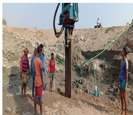
Figure 3-66: Executing the sand pile for DS-3/4 of Polder 48
