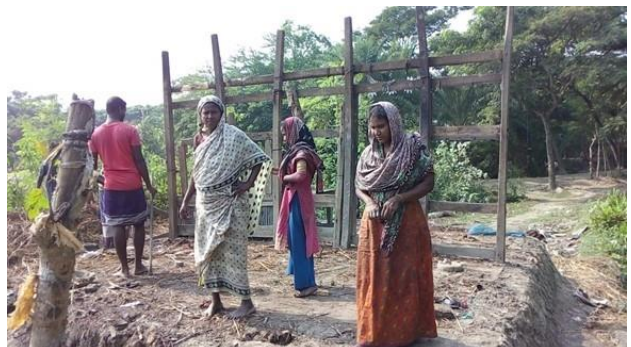
Figure 3-16: Removing house for construction of FS-1 in Polder 35/3
