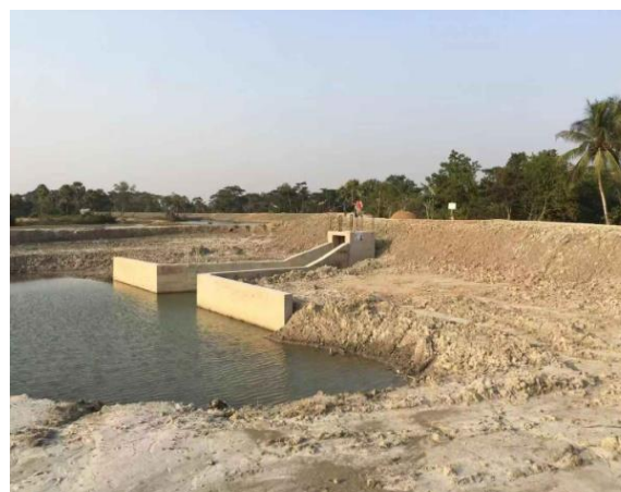
Figure 3-64: Site view of complete sluice-FS- 7 of Polder-47/2
