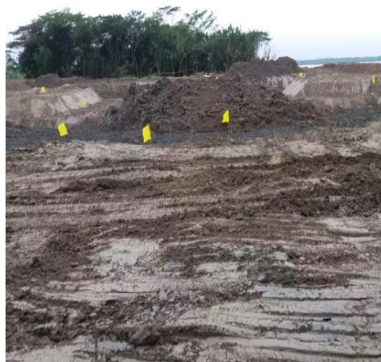
Figure 3-56: Excavating the Foundation for the DS-7 of Polder 39/2C
