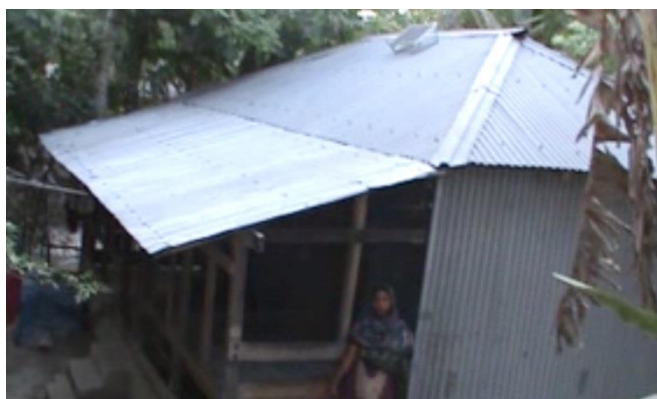
HHs ID 123 Resident Structure Before Relocation Polder No. 35/1
