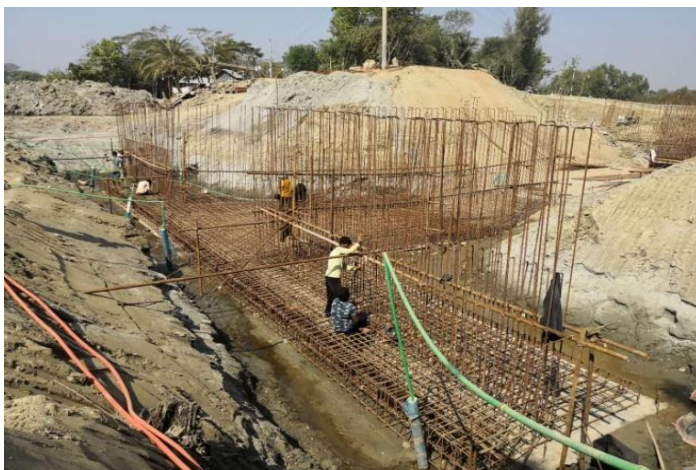
Figure 3-65: Fitting the deformed bar for DS-3/4 of Polder-48
