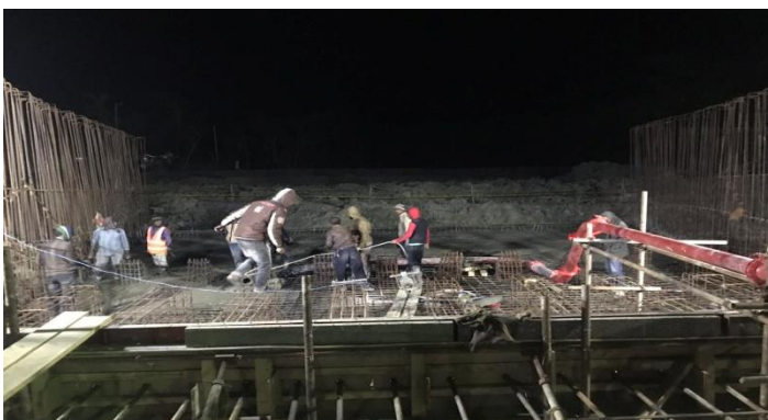
Figure 3-59: Pouring the RCC slab for DS-5 nighttime of Polder-41/1
