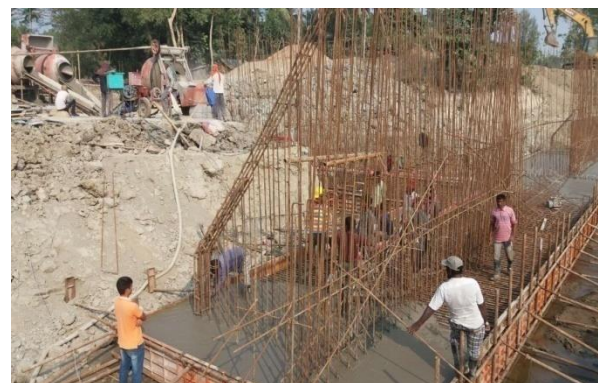
Figure 3-60: Pouring the RCC slab for DS-8 of Polder-41/1
