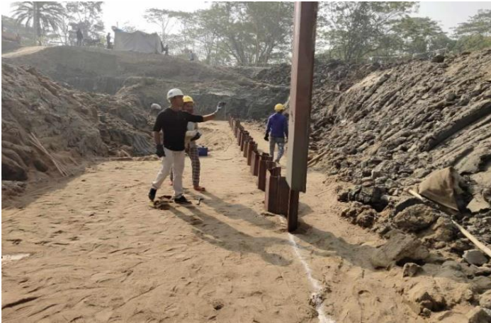
Figure 3-61: Driving the sheet pile for DS-9 of Polder-41/1
