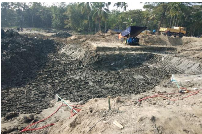
Figure 3-63: Dewatering for DS-7 of Polder 43/2C
