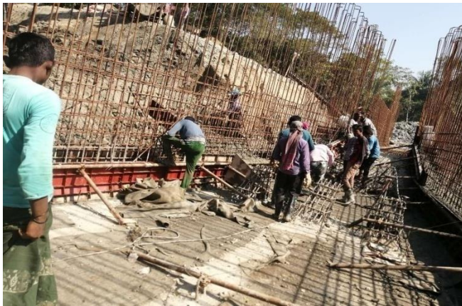
Figure 3-57: Fitting the deformed bar for DS-2 of Polder-40/2
