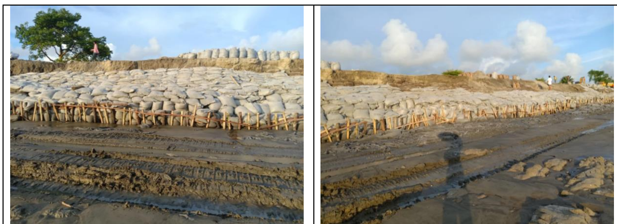
Figure 3-71: Emergency Work of Polder-48
