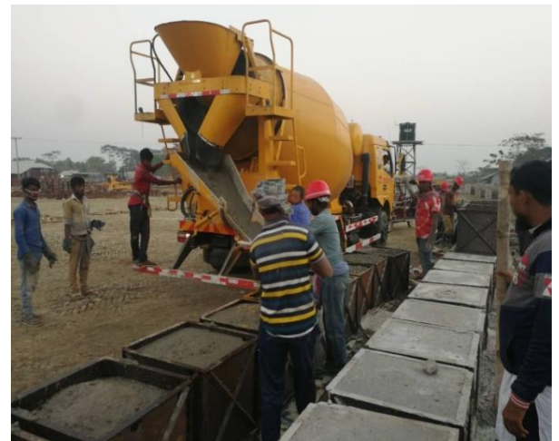
Figure 3-66: Manufactured the new size (60*60*60cm) block in yard No.1 of Polder-48
