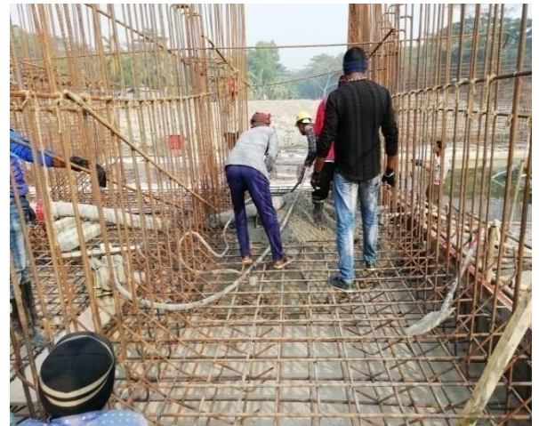
Figure 3-62: Pouring the RCC slab for DS-5 daytime of Polder-41/1
