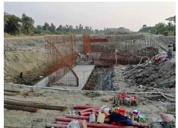
Figure 3-64: Pouring the RCC slab for DS-1 in Polder-47/2
