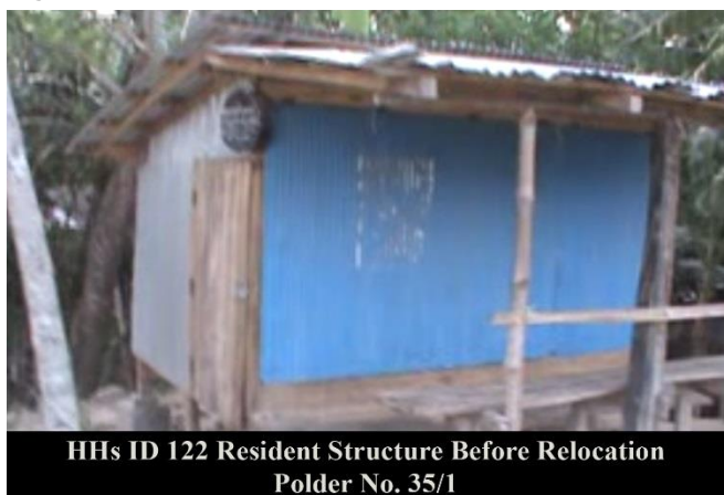
Figure 3-9: HH 122 Before relocation of Polder-35/1
