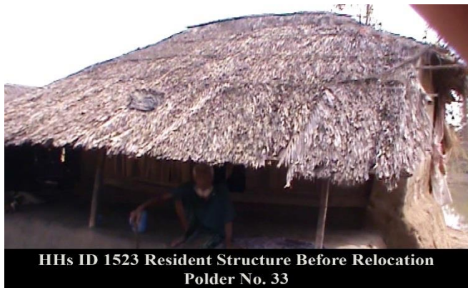
Figure 3-5: HH 1523 Before relocation of Polder-33
