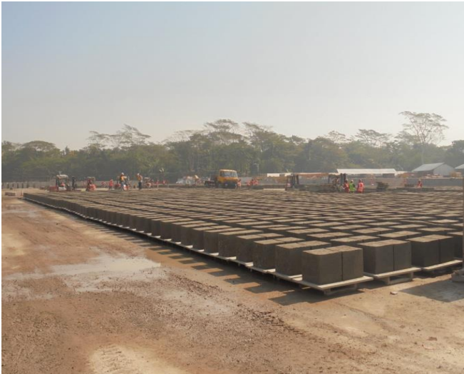
Figure 3-55: Curing the blocking yard no.1 of Polder-39/2C
