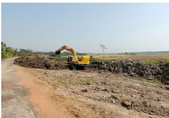
Figure 3-69: EMB construction around KM 9+700 of Polder-41/1
