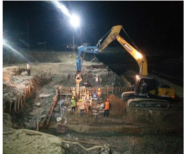
Figure 3-56: Executing the sand pile for DS-07 of Polder-39/2C
