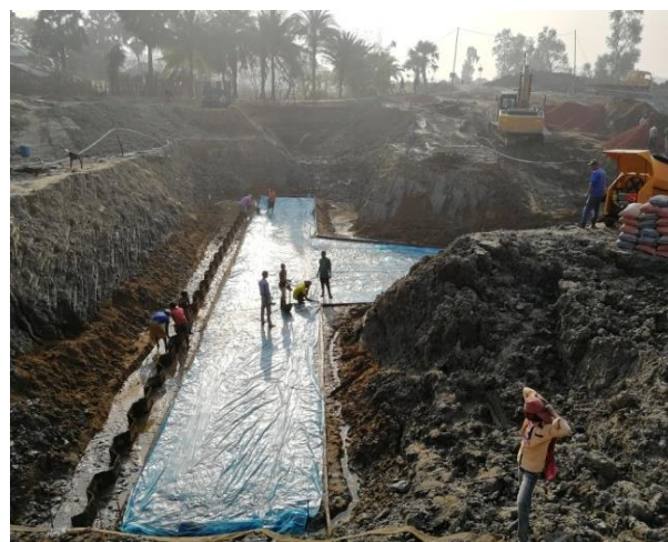
Figure 3-68: Pouring the lean concrete for DS-3 of Polder-47/2
