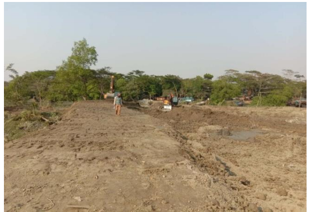
Figure 3-58: Excavating the foundation for DS-4/5 of Polder-40/2
