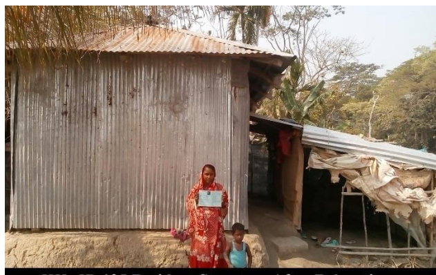
HHs ID 125 Resident Structure After Relocation Polder No. 35/1
