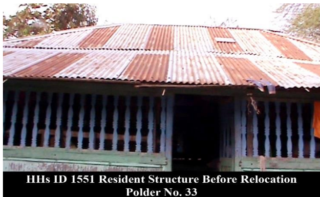
Figure 3-7: HH 1551 Before relocation of Polder-33
