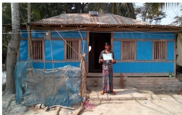
HHs ID 123 Resident Structure After Relocation Polder No. 35/1
