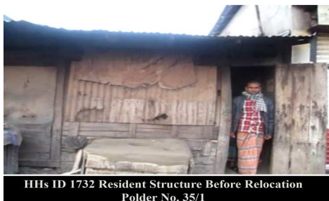
Figure 3-17: HH 1732 Before relocation of Polder-35/1
