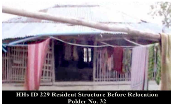
Figure 3-9: HH 229 Before relocation of Polder-32
