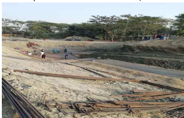
Figure 3-63: Pouring the lean concrete for FS-10 of Polder-40/2
