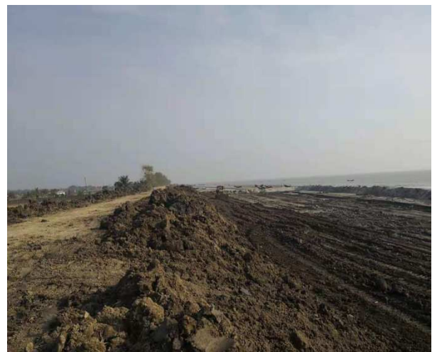
Figure 3-74: Spreading the materials for EBM construction around
