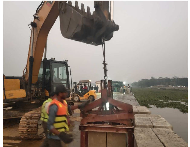
Figure 3-60: Loading the CC blocks for bank protection work of Polder-39/2C
