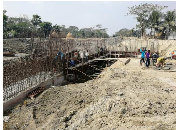
Figure 3-72: Pouring the RCC wall for DS-2 of Polder-47/2
