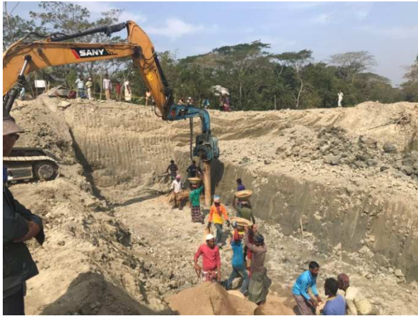
Figure 3-65: Executing the sand pile for DS-6 of Polder-41/1
