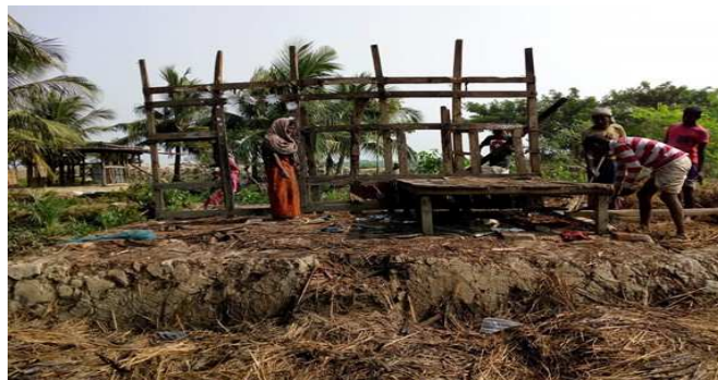
Figure 3-19: House relocation at FS-1 in Polder 35/3
