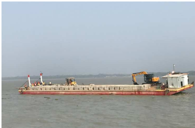
Figure 3-61: Transporting the CC blocks for bank protection work of Polder-39/2C
