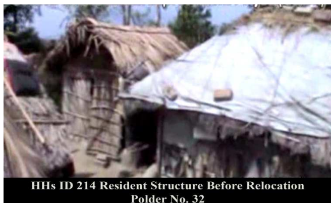
Figure 3-11: HH 214 Before relocation of Polder-32
