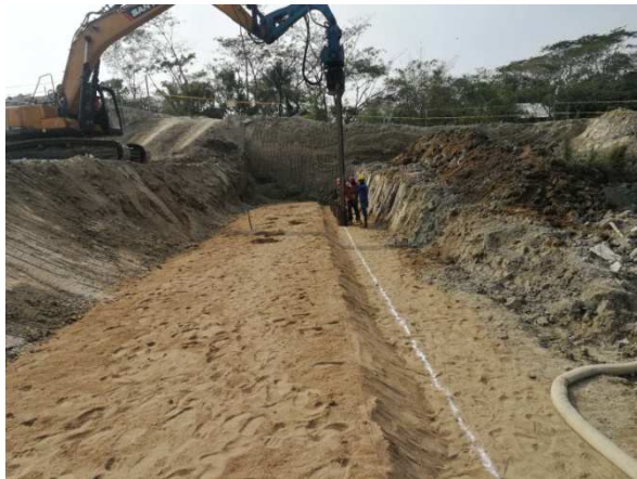
Figure 3-67: Driving the sheet pile for DS-6 of Polder-41/1
