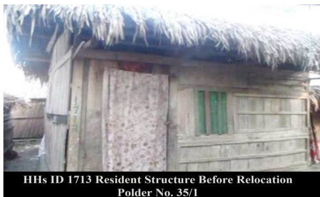
Figure 3-15: HH 1713 Before relocation of Polder-35/1
