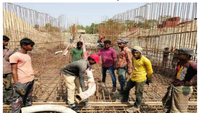
Figure 3-64: Pouring the RCC slab for FS-10 of Polder-40/2
