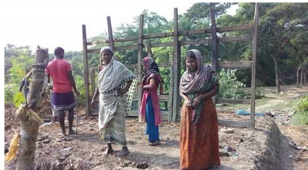
Figure 3-20: Removing house for construction of FS-1 in Polder 35/3
