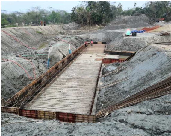
Figure 3-69: Establishing the LC form for DS-7 of Polder-43/2C
