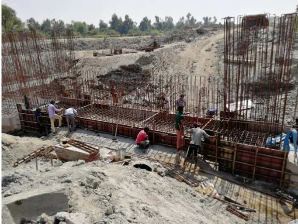
Figure 3-71: Establishing the RCC form for DS-1 of Polder-47/2
