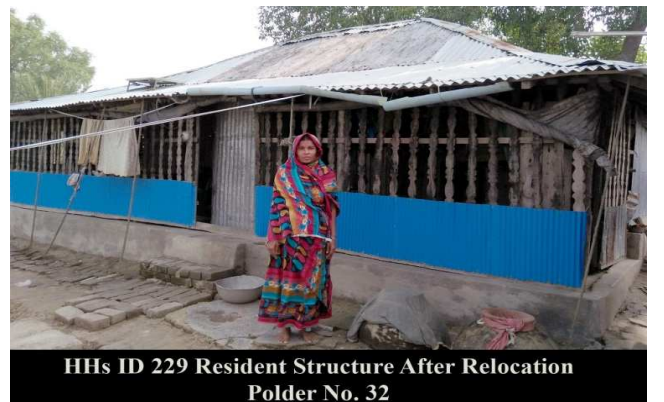
Figure 3-10: HH 229 After relocation of Polder-32
