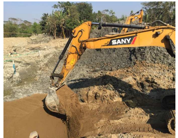
Figure 3-70: Sand filling for the foundation for DS-07 of Polder-43/2C
