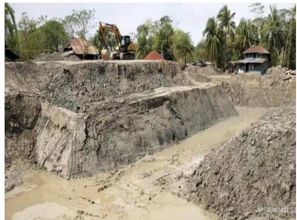
Figure 3-62: Excavating the foundation for FS-9 of Polder-40/2
