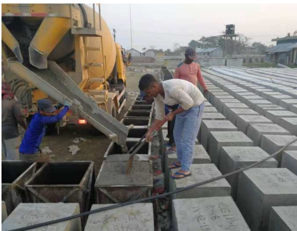
Figure 3-73: Making the CC block in yard no. 1 of Polder-48
