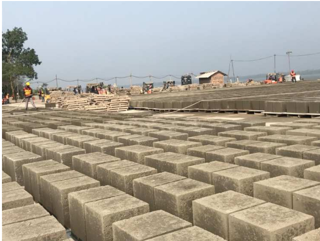
Figure 3-59: Curing the blocking yard no.2 of Polder-39/2C
