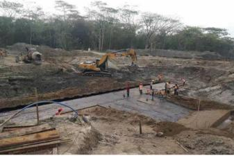
Figure 3-60: Pouring the Lean Concrete For DS-7 of Polder-39/2C
