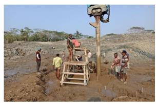
Figure 3-62: Executing the Sand Pile For DS-5 of Polder-40/2
