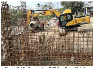
Figure 3-65: Pouring the RCC Box Base Slab For DS-9 of Polder-41
