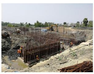
Figure 3-69: Establishing the Form for RCC Wall for DS-3 of Polder-47/2
