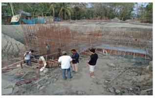
Figure 3-63: Fixing the Deformed Bar For FS-10 of Polder-40/2
