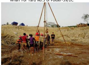
Figure 3-61: Drilling the Dewatering Bore Hole For DS-5 of Polder-40/2
