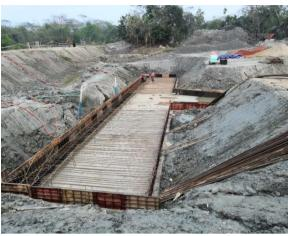
Figure 3-68: Establishing the LC form for DS-7 of Polder-43/2C
