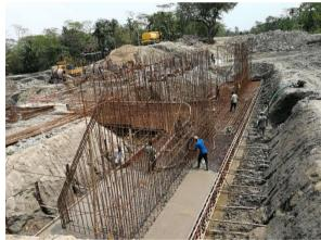
Figure 3-67: Pouring the RCC Base Slab For DS-6 of Polder-41/1
