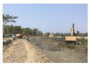
Figure 3-71: Excavating the Drainage Channel Near DS-3-4 of Polder-47/2
