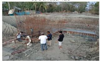
Figure 3-67: Fixing the Deformed Bar For FS-10 of Polder-40/2
