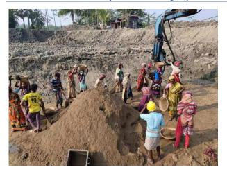
Figure 3-68: Executing the Sand Pile for DS-7of Polder-41/1
