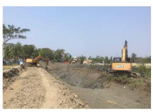
Figure 3-75: Excavating the Drainage Channel Near DS-3-4 of Polder-47/2
