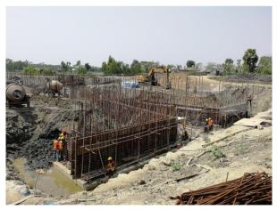
Figure 3-73: Establishing the Form for RCC Wall for DS-3 of Polder-47/2
