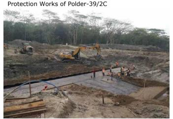
Figure 3-64: Pouring the Lean Concrete For DS-7 of Polder-39/2C
