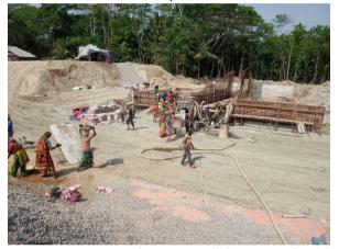
Figure 3-70: Pouring the RCC Wall for FS-1 of Polder-
