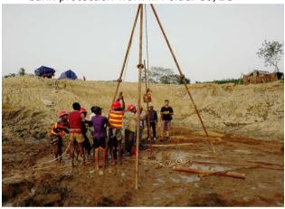
Figure 3-65: Drilling the Dewatering Bore Hole For DS-5 of Polder-40/2
