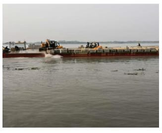
Figure 3-63: CC Blocks dumping for river bank protection work in Polder 39/2C
