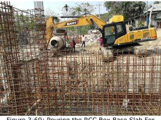
Figure 3-69: Pouring the RCC Box Base Slab For DS-9 of Polder-41
