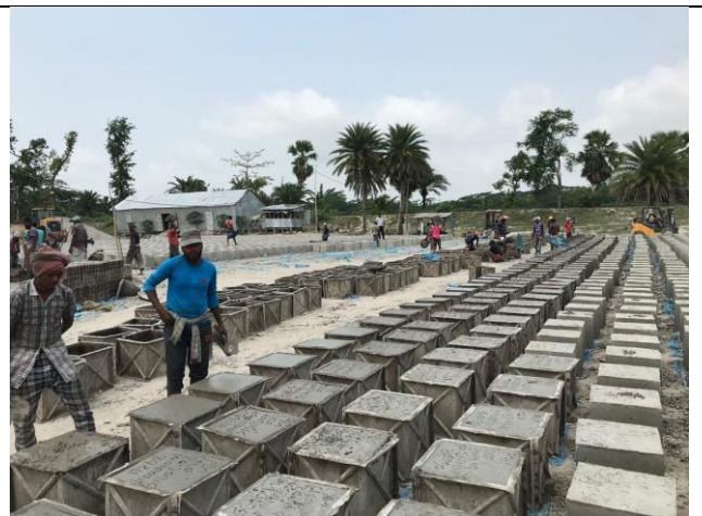
Figure 3-67: CC Blocks manufacturing at yard #2 (KM13+000) in Polder 41/1
