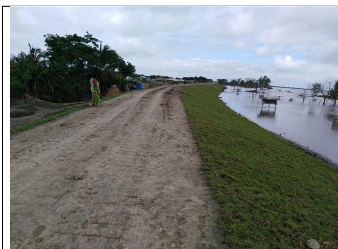
Figure 3-41: Completed Embankment in Polder-32
