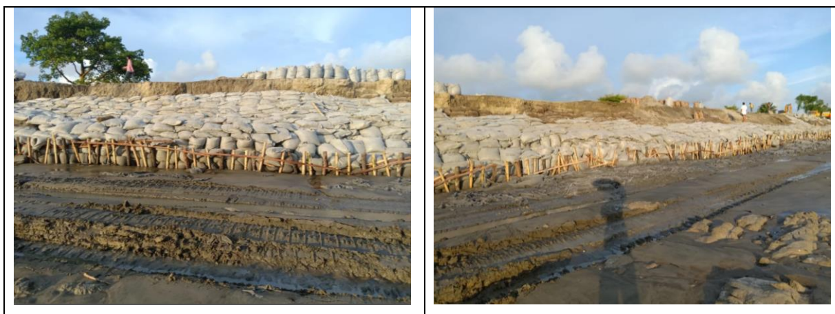
Figure 3-80: Emergency Work of Polder-48
