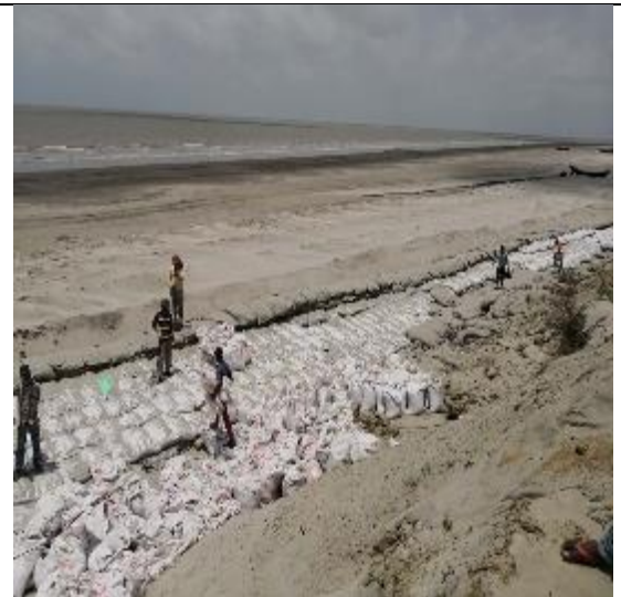
Figure 3-79: Synthetic bags placing for emergency slope protection work 31+280-31+408 in Polder 48
