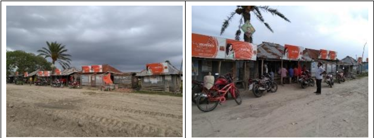
Figure 3-19: Relocation site at Mollikerber Madrasha Bazar in Polder-35/3
