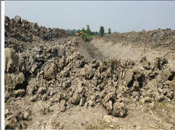
Figure 3-68: Excavation / Re-sectioning for drainage channel of DS-04 (KM0+000-0+260) in Polder 41/1
