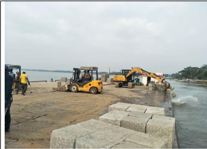
Figure 3-62: CC Blocks dumping for slope protection work (KM51+041-53+418) in Polder 39/2C
