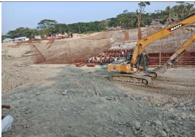
Figure 3-66: Form work for end sill of DS-05 in Polder 40/2
