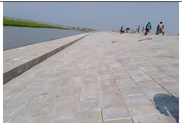
Figure 3-46: Completed Slope Protection Works in Polder-32
