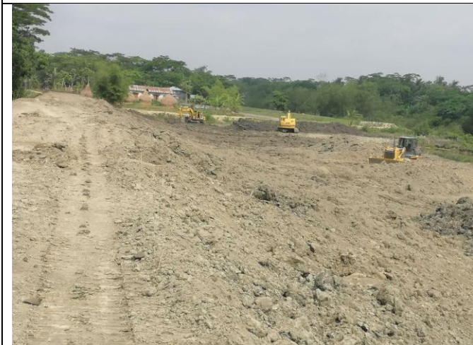
Figure 3-70: Earth work for embankment KM0+900-1+300 in Polder 43/2C
