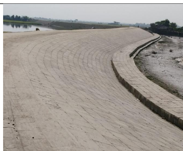
Figure 3-42: Completed Slope Protection Works in Polder-32
