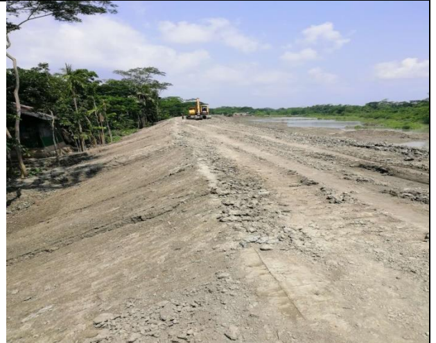
Figure 3-69: Earth Work for Embankment KM1+000 to Km2+000 in Polder 43 /2C
