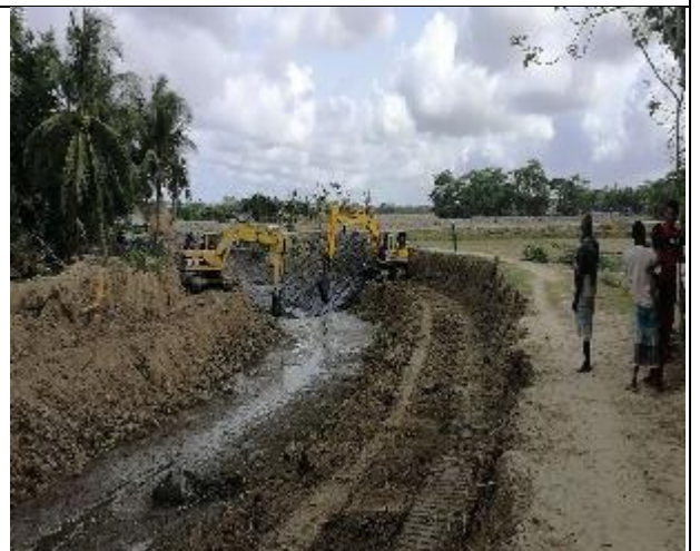
Figure 3-73: Excavation / Re-sectioning for drainage channel of DS-03 in Polder 47/2
