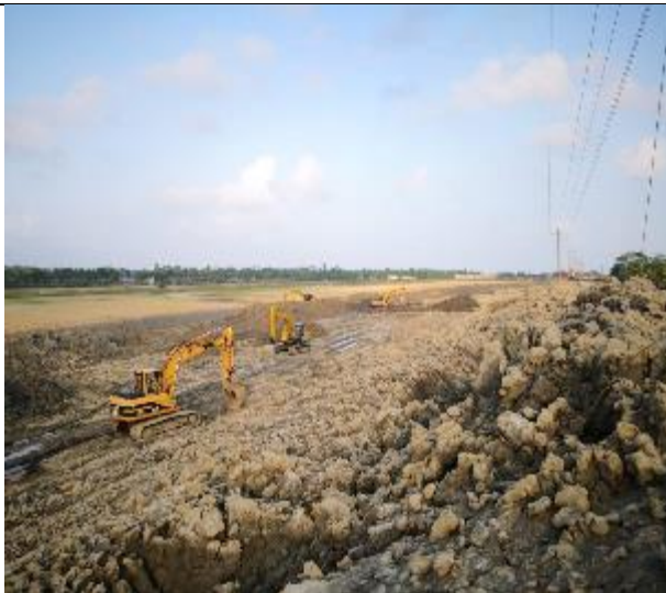
Figure 3-78: Earth work for embankment KM16+134-17+000 in Polder 48
