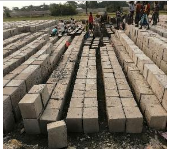
Figure 3-75: CC Blocks manufacturing at yard #1 (KM7+000) in Polder 47/2
