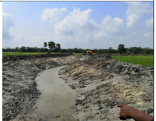
Figure 3-71: Excavation / Re-sectioning for drainage channel of DS-07 (KM0+000-2+440) in Polder 43/2C
