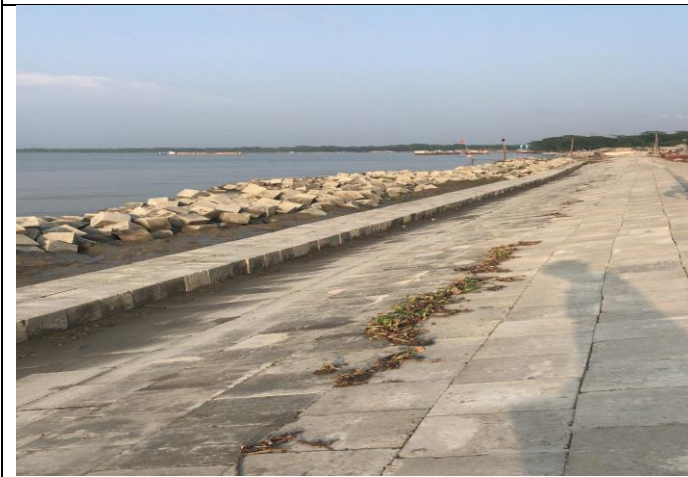
Figure 3-64: Completed section of slope protection work (KM51+041-53+418) in Polder 39/2C
