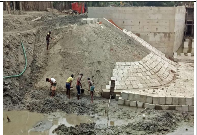
Figure 3-65: Placing of CC block for DS-03 in Polder 40/2
