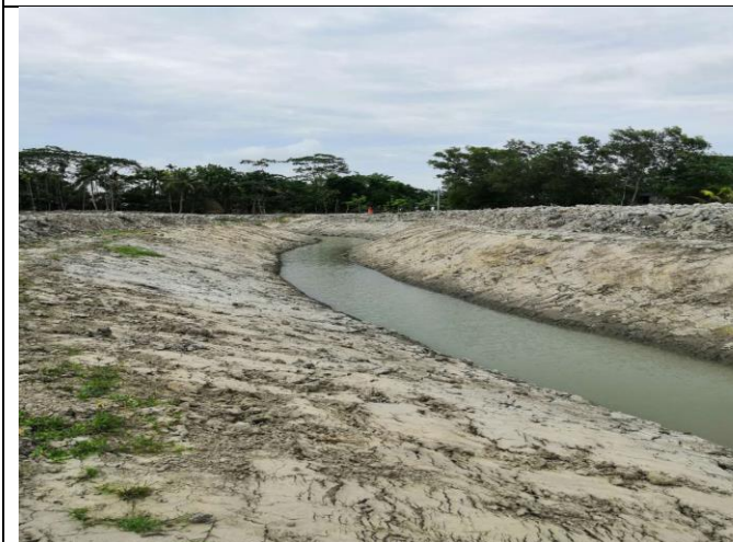
Figure 3-72: Completed Section Drainage Channel for DS-07 in Polder 43/2C
