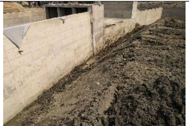
Figure 3-77: Back filling for DS-01 in Polder 48
