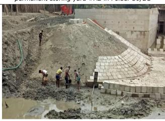
Figure 3-65: Placing of CC block for DS-03 in Polder 40/2
