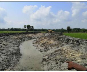
Figure 3-71: Excavation / Re-sectioning for drainage channel of DS-07 (KM0+000-2+440) in Polder 43/2C
