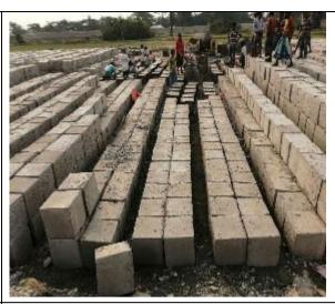
Figure 3-75: CC Blocks manufacturing at yard #1 (KM7+000) in Polder 47/2
