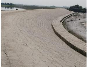
Figure 3-42: Completed Slope Protection Works in Polder-32
