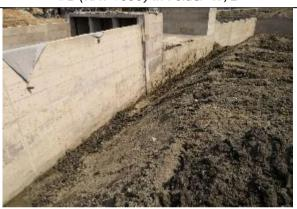
Figure 3-77: Back filling for DS-01 in Polder 48
