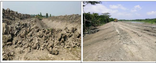
Figure 3-68: Excavation / Re-sectioning for drainage channel of DS-04 (KM0+000-0+260) in Polder 41/1
