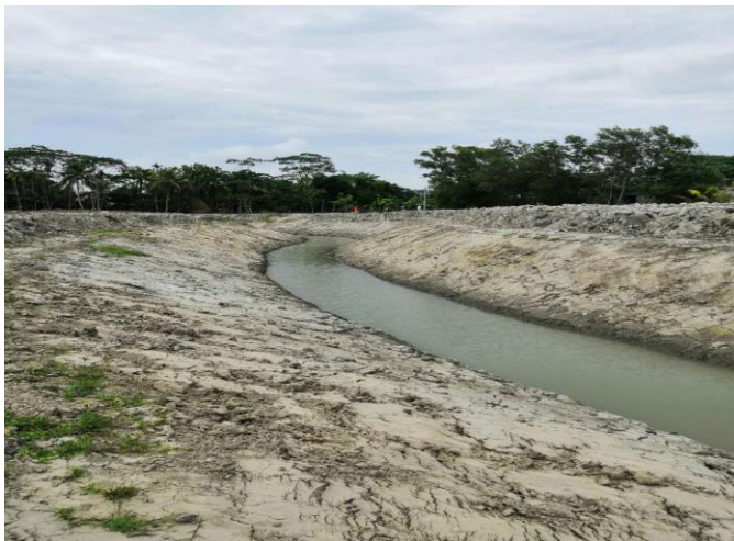
Figure 3-67: Completed Section Drainage Channel for DS-07 in Polder 43/2C
