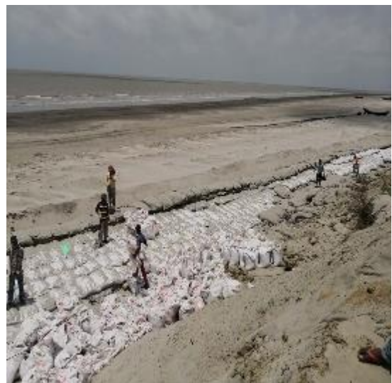
Figure 3-74: Synthetic bags placing for emergency slope protection work 31+280-31+408 in Polder 48
