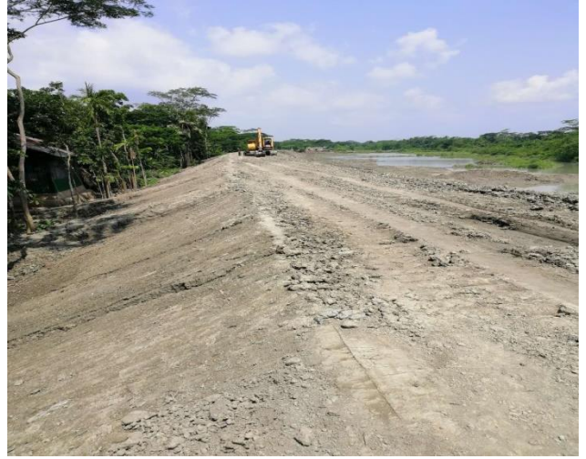
Figure 3-64: Earth Work for Embankment KM1+000 to Km2+000 in Polder 43 /2C
