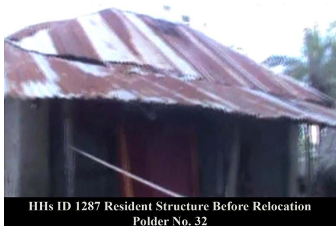
Figure 3-1: HH 1287 Before relocation of Polder-32
