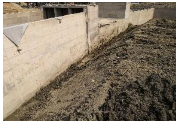
Figure 3-72: Back filling for DS-01 in Polder 48
