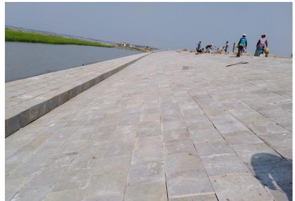
Figure 3-39: Completed Slope Protection Works in Polder-32
