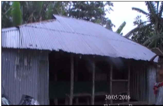
HH ID 226 Resident Structure before Relocation
