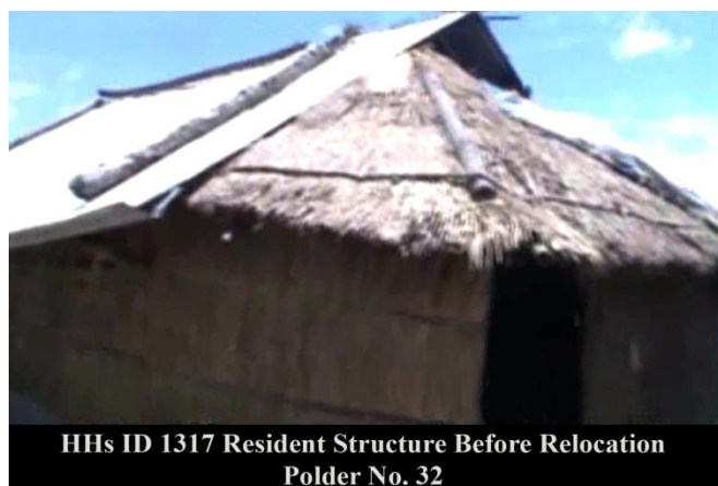
Figure 3-3: HH 1317 Before relocation of Polder-32
