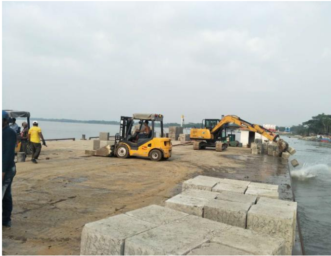
Figure 3-57: CC Blocks dumping for slope protection work (KM51+041-53+418) in Polder 39/2C
