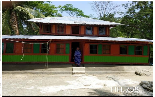
HH ID 758 Resident Structure After Relocation
