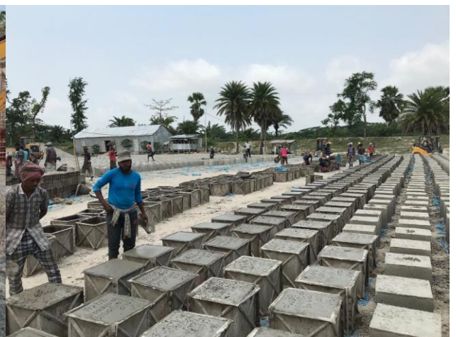
Figure 3-62: CC Blocks manufacturing at yard #2 (KM13+000) in Polder 41/1
