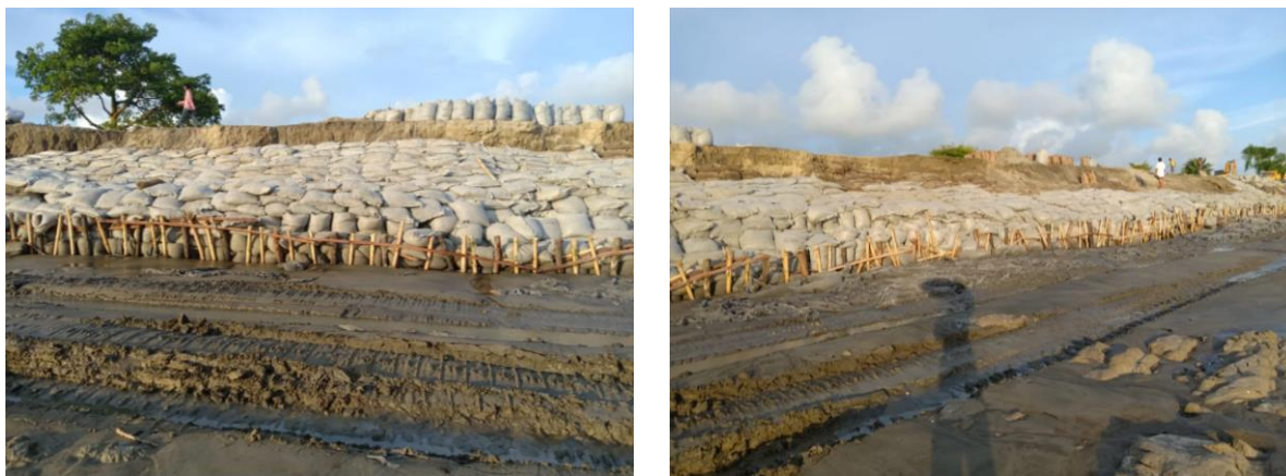
Figure 3-75: Emergency Work of Polder-48
