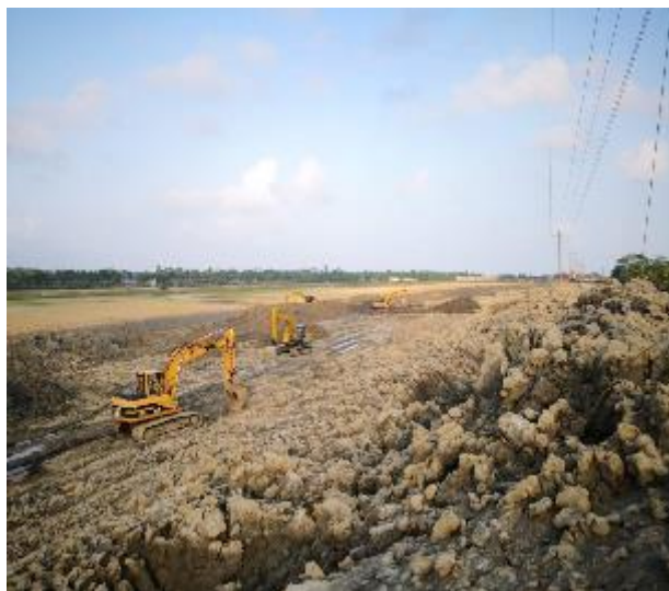
Figure 3-73: Earth work for embankment KM16+134-17+000 in Polder 48
