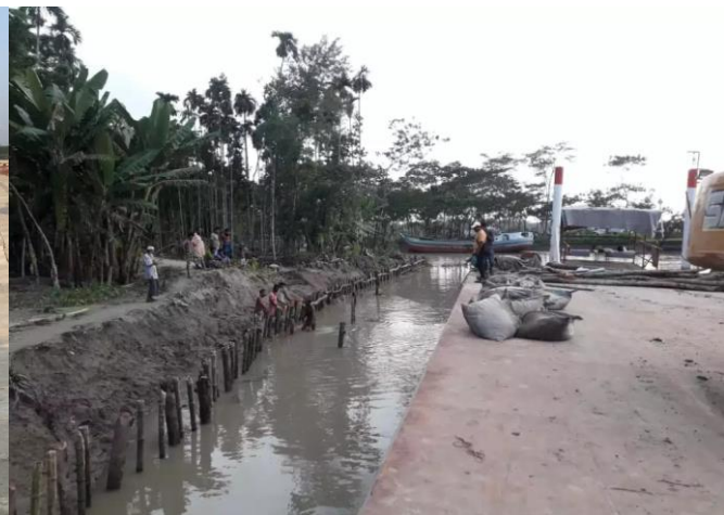
Figure 3-60: Emergency Temporary bank protection work in Polder-39/2C
