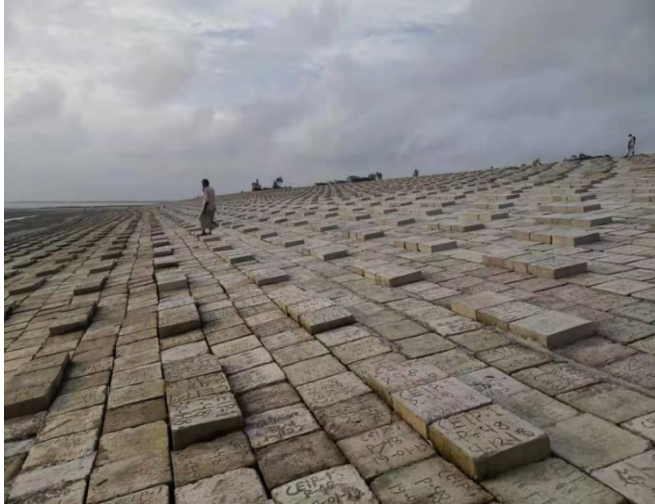
Figure 3-63: Site View of Slope Protection work of Polder 48
