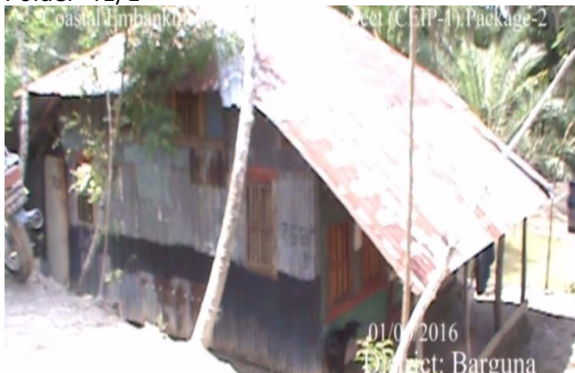
HH ID 758 Resident Structure before Relocation
