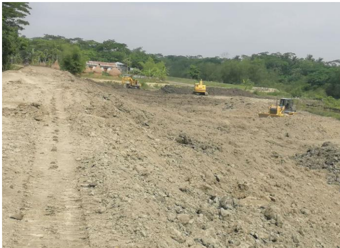
Figure 3-65: Earth work for embankment KM0+900-1+300 in Polder 43/2C
