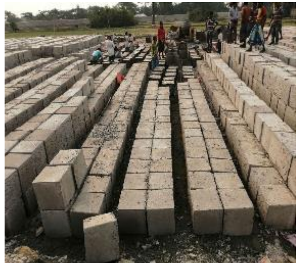
Figure 3-70: CC Blocks manufacturing at yard #1 (KM7+000) in Polder 47/2
