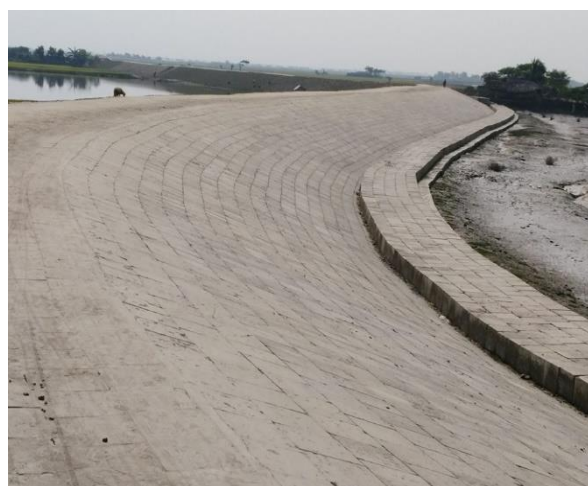
Figure 3-35: Completed Slope Protection Works in Polder-32
