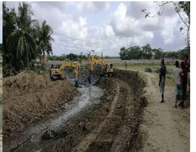
Figure 3-68: Excavation / Re-sectioning for drainage channel of DS-03 in Polder 47/2
