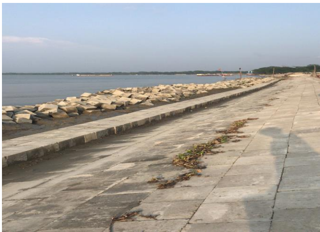
Figure 3-59: Completed section of slope protection work (KM51+041-53+418) in Polder 39/2C
