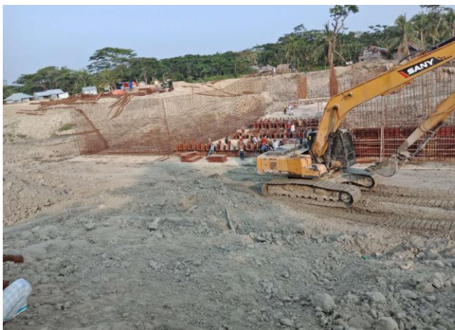
Figure 3-61: Form work for end sill of DS-05 in Polder 40/2
