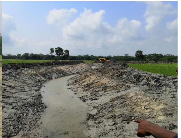
Figure 3-66: Excavation / Re-sectioning for drainage channel of DS-07 (KM0+000-2+440) in Polder 43/2C
