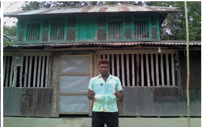
HH ID 226 Resident Structure after Relocation
