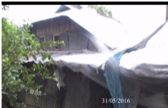
HH's No 415 Resident Structure Before Relocation Polder 41/1
