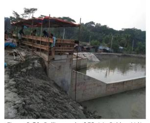
Figure 3-56: Ralling work of FS-1 in Polder-41/1
