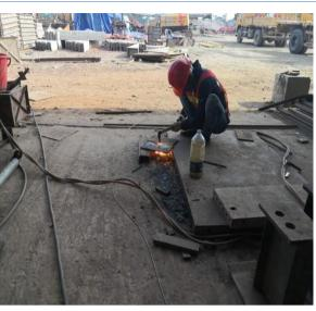
Figure 3-65: Repair formwork for CC block in Polder 48
