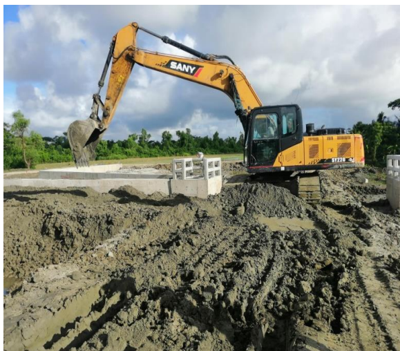
Figure 3-62: Back fill & Repair of access road for DS-01 in Polder 47/2
