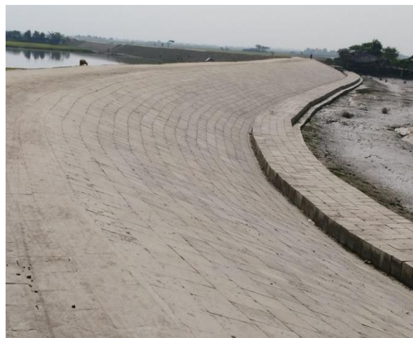
Figure 3-34: Completed Slope Protection Works in Polder-32
