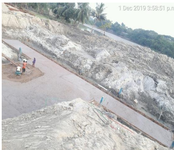
Figure 3-67: DS-3/3 CC casting at CS in Polder-48
