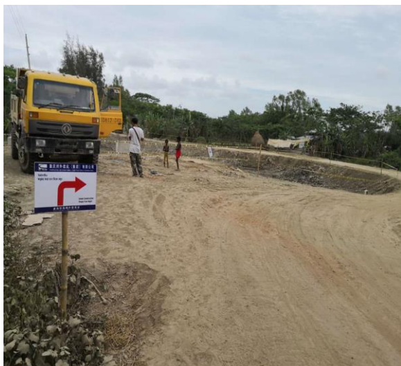
Figure 3-64: Install of Waring Tape for FS-3 in Polder 48
