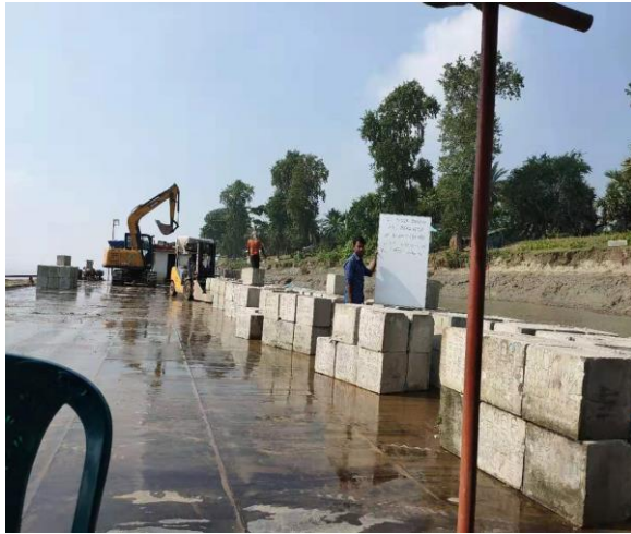
Figure 3-58: Dumping work in Polder-41/1
