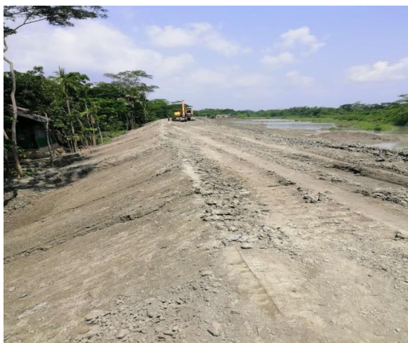
Figure 3-60: Earth Work for Embankment KM1+000 to Km2+000 in Polder 43 /2C
