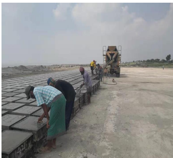
Figure 3-66: CC Block Manufacturing in Polder 48 at yard-3
