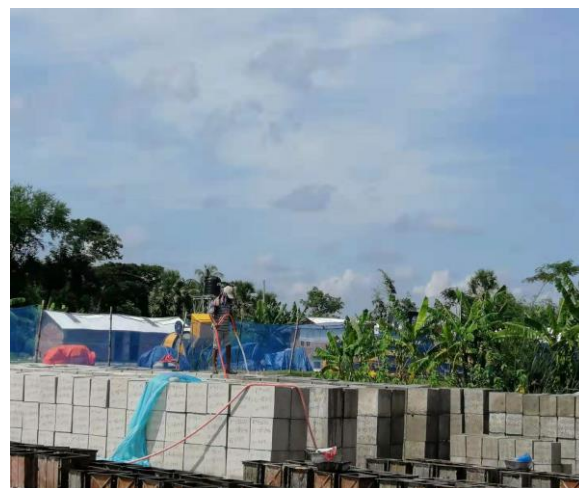
Figure 3-61: Curing CC Blocks in Polder 43/2C at DS-1 yard
