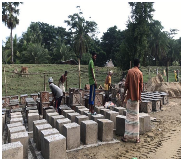
Figure 3-63: CC block manufacturing in Polder 47/2 at yard-1
