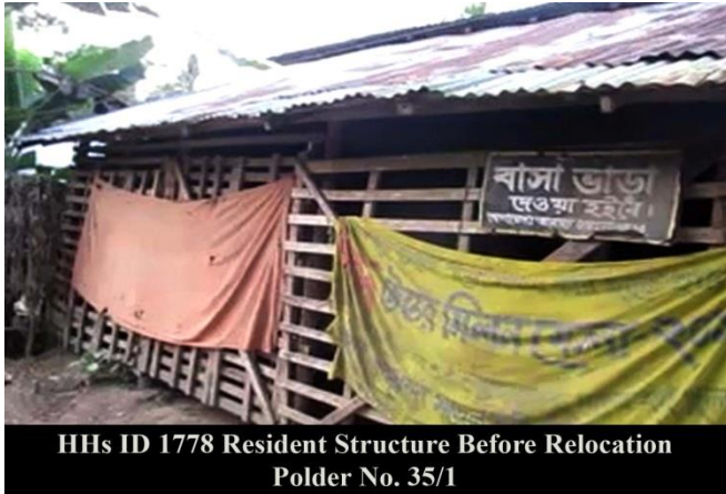
HHs ID 1778 Resident Structure Before Relocation Polder No. 35/1
