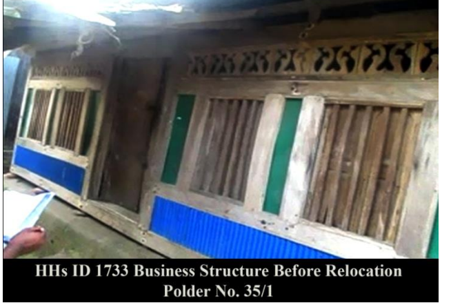
HHs ID 1733 Business Structure Before Relocation Polder No. 35/1
