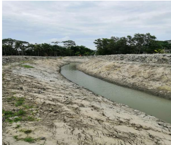
Figure 3-59: Completed Section Drainage Channel for DS-07 in Polder 43/2C
