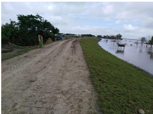
Figure 3-33: Completed Embankment in Polder-32
