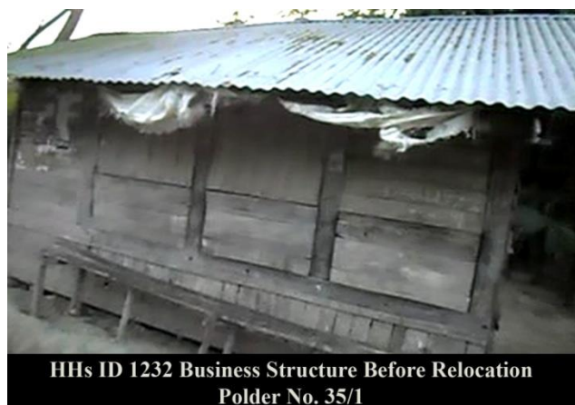
Figure 3-3: HH1232 Before relocation of Polder-35/1
