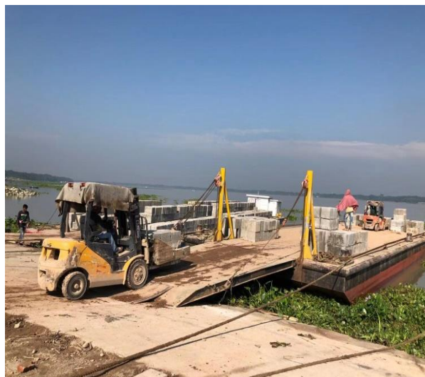
Figure 3-65: Loading CC Block on the berge in Polder 39-2C
