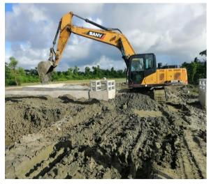
Figure 3-62: Back fill& Repair of access road for DS-01 in Polder 47/2
