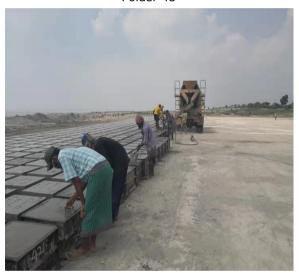
Figure 3-66: CC Block Manufacturing in Polder 48 at yard-3
