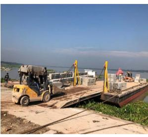
Figure 3-65: Loading CC Block on the berge in Polder 39-2C
