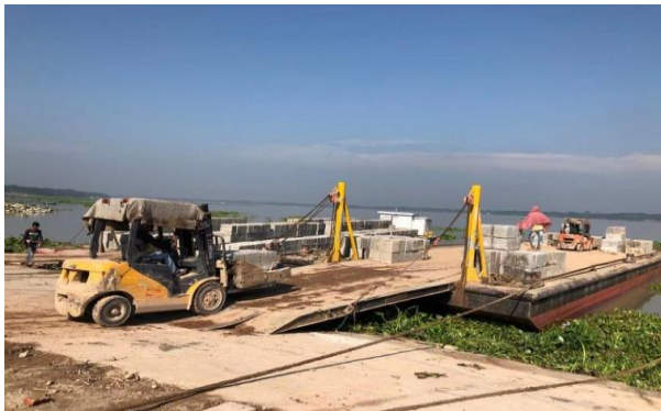
Figure 3-70: Loading CC Block on the barge in Polder 39-2C
