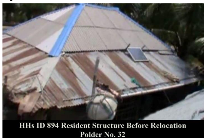
Figure 3-3: HH 894 Before relocation of Polder-32
