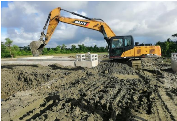
Figure 3-67: Back fill & Repair of access road for DS-01 in Polder 47/2
