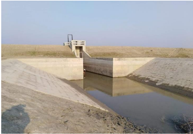
Figure 3-40: Completed DS of Polder-32
