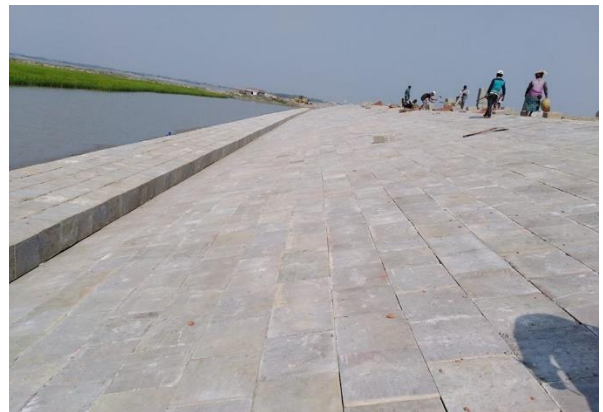
Figure 3-43: Completed Slope Protection Works in Polder-32
