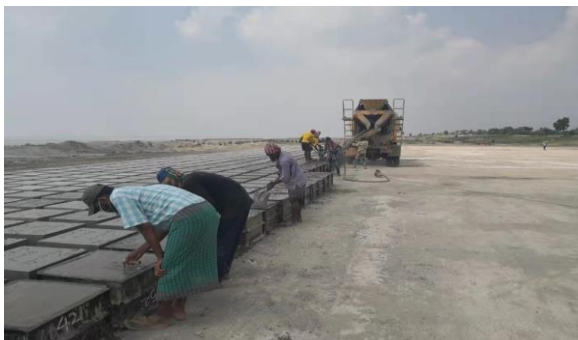
Figure 3-71: CC Block Manufacturing in Polder 48 at yard-3
