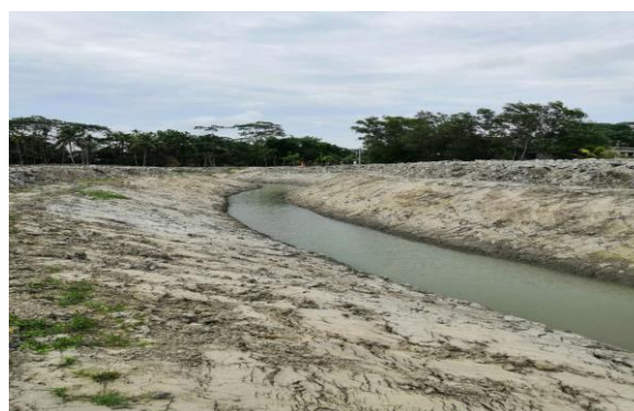
Figure 3-64: Completed Section Drainage Channel for DS-07 in Polder 43/2C
