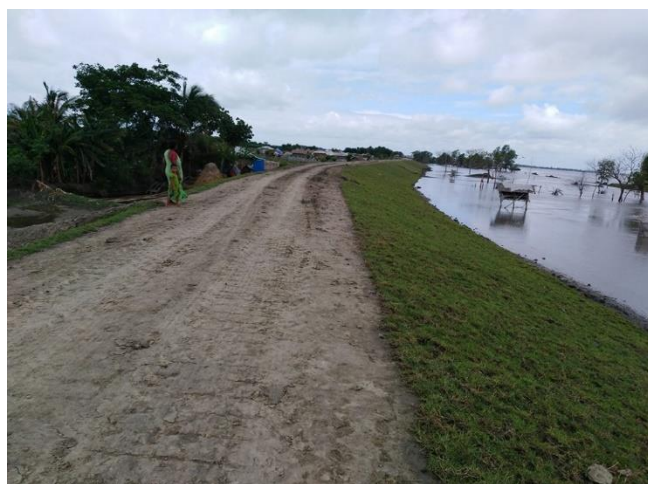
Figure 3-38: Completed Embankment in Polder-32
