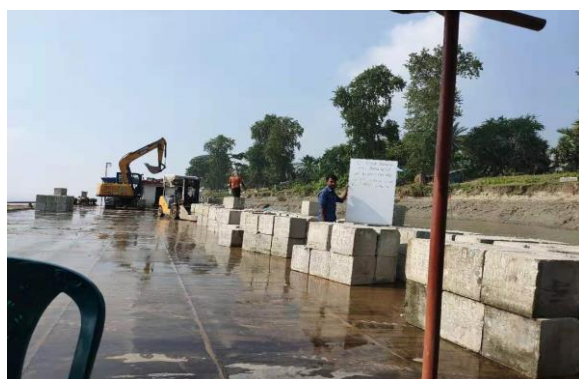
Figure 3-63: Dumping work in Polder-41/1
