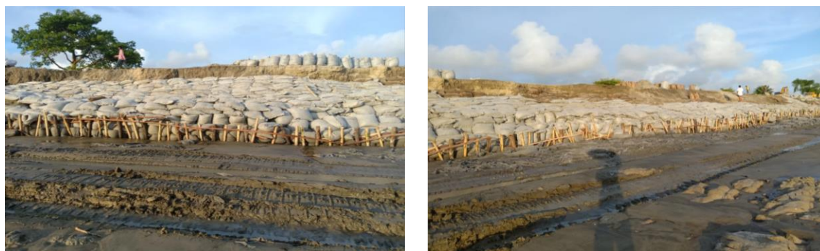
Figure 3-73: Emergency Work of Polder-48
