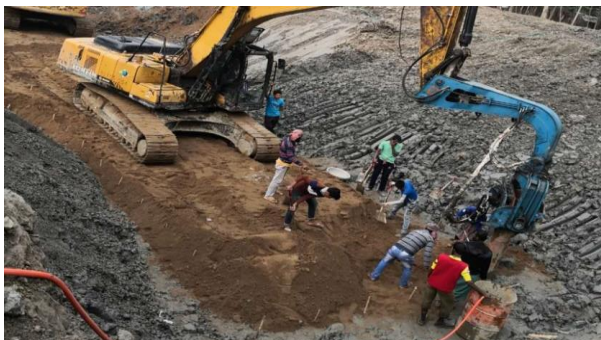
Figure 3-72: Sand pile work for DS-8 in Polder 43-2C
