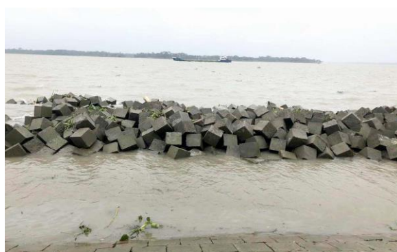
Figure 3-61: Dumping the CC Block at Km 51 in Polder 39-2C
