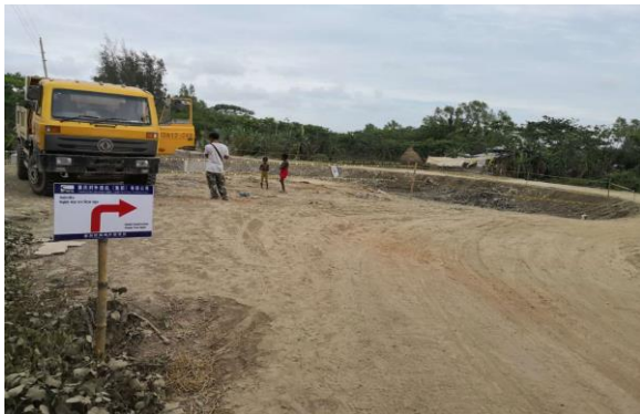
Figure 3-69: Install of Warning Tape for FS-3 in Polder 48
