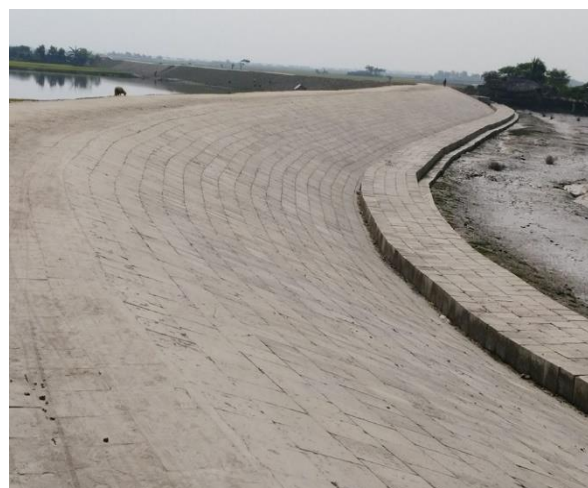
Figure 3-39: Completed Slope Protection Works in Polder-32
