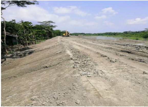
Figure 3-65: Earth Work for Embankment KM1+000 to Km2+000 in Polder 43 /2C
