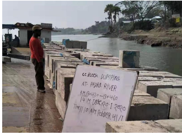
Figure 3-66: Dumping the CC Block at Km 13 in Polder 41-1
