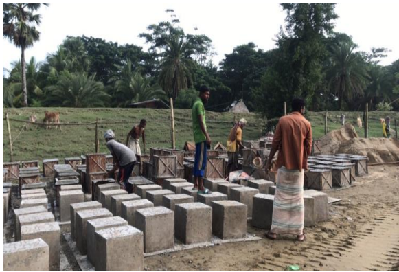
Figure 3-68: CC block manufacturing in Polder 47/2 at yard-1
