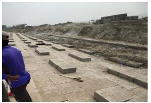
Figure 3-42: Slope Protection work in Polder 48
