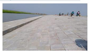
Figure 3-17: Completed Slope Protection Works in Polder-32
