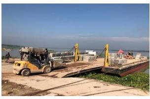
Figure 3-44: Loading CC Block on the berge in Polder-39/2C
