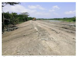
Figure 3-39: Finishing Work for Embankment in Polder 43 /2C
