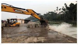
Figure 3-36: Dumping CC Block for river bank protection work (KM51+041-53+418) in Polder 39-2C
