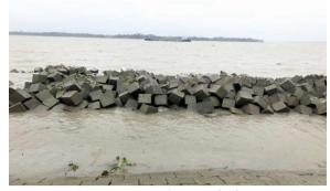
Figure 3-35: Dumping the CC Block at Km 51 in Polder 39-2C
