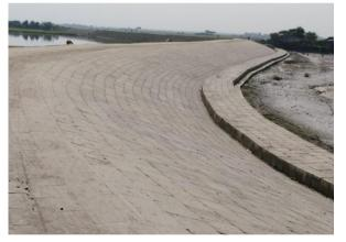
Figure 3-13: Completed Slope Protection Works in Polder-32
