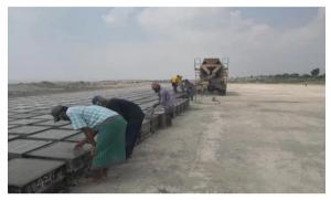
Figure 3-45: CC Block Manufacturing in Polder 48 at yard-3
