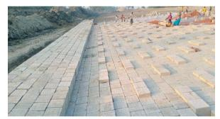
Figure 3-35: Ongoing Slope Protection Works (Polder 40/2), Barguna
