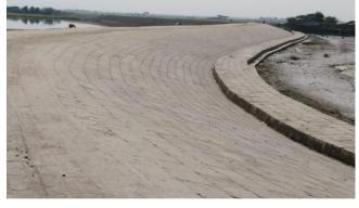
Figure 3-13: Completed Slope Protection Works in Polder-32
