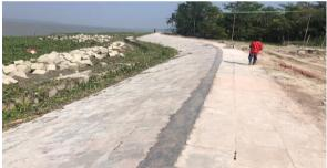
Figure 3-36: Bank Protection with Pitching Works (Polder 39/2C)
