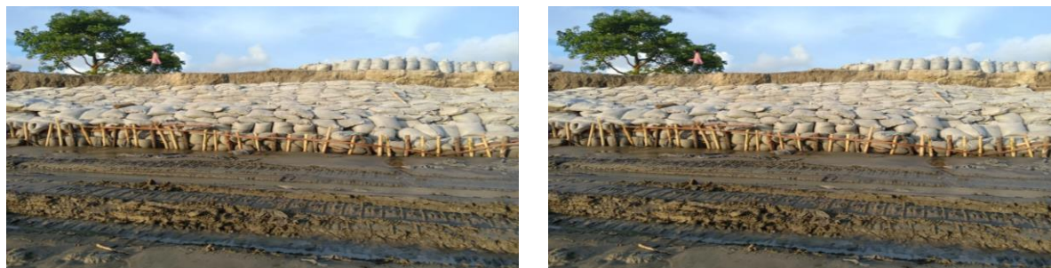
Figure 3-39: Emergency Work in Polder-48
