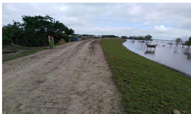
Figure 3-12: Completed Embankment in Polder-32
