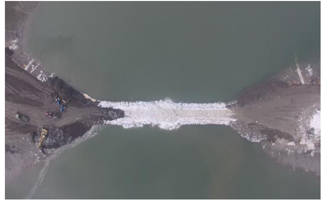
Figure 3-19: Nalian Closure Dam of Polder-32 (ongoing)
