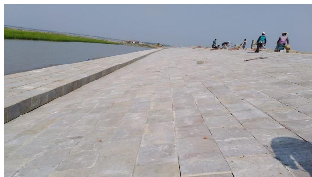
Figure 3-17: Completed Slope Protection Works in Polder-32
