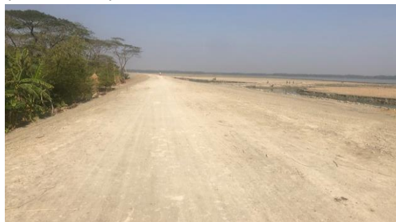
Figure 3-38: Completed Embankment CEIP-1, W/02, Polder 43/2C
