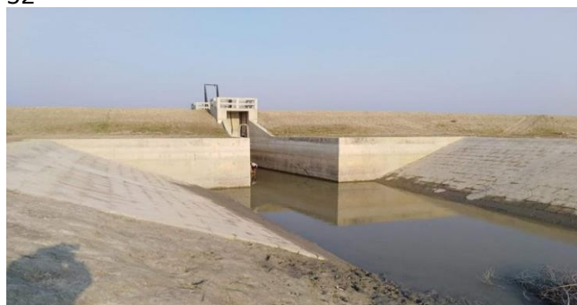
Figure 3-14: Completed DS of Polder-32
