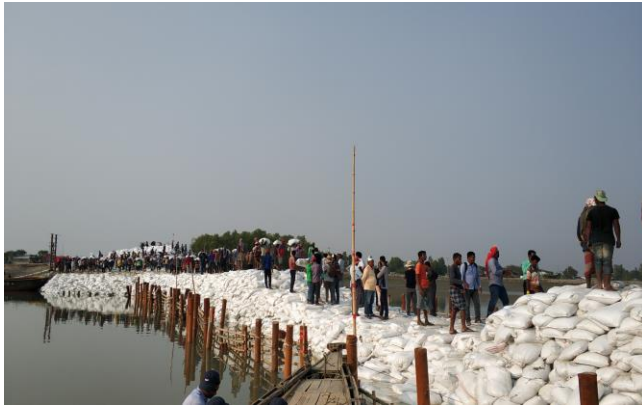
Figure 3-18: Nalian Closure Dam of Polder-32 (ongoing)
