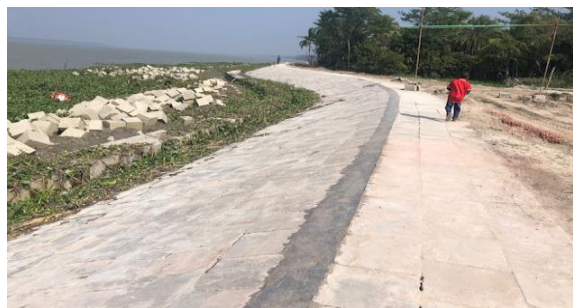
Figure 3-36: Bank Protection with Pitching Works (Polder 39/2C)
