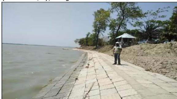
Figure 3-37: Ongoing Bank Protection in Polder-41/1
