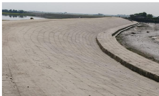
Figure 3-13: Completed Slope Protection Works in Polder-32
