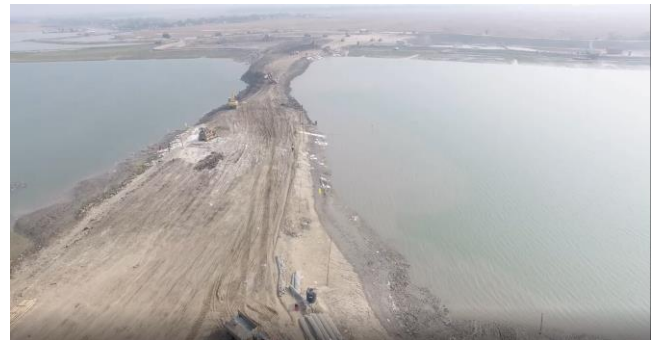
Figure 3-21: Nalian Closure Dam of Polder-32 (ongoing)
