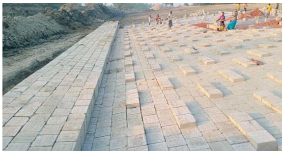
Figure 3-35: Ongoing Slope Protection Works (Polder 40/2), Barguna
