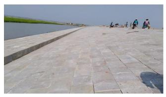
Figure 3-14: Completed Slope Protection Works in Polder-32
