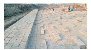
Figure 3-31: Ongoing Slope Protection Works (Polder 40/2), Barguna
