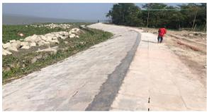
Figure 3-32: Bank Protection with Pitching Works (Polder 39/2C)
