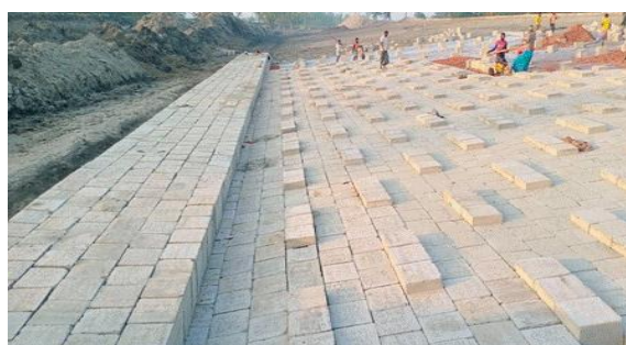
Figure 3-27: Ongoing Slope Protection Works (Polder 40/2), Barguna
