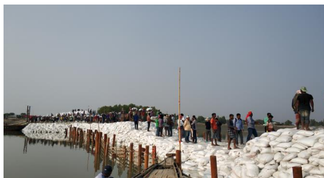
Figure 3-11: Nalian Closure Dam of Polder-32 (ongoing)
