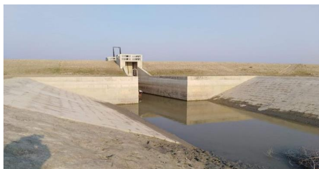
Figure 3-9: Completed DS of Polder-32
