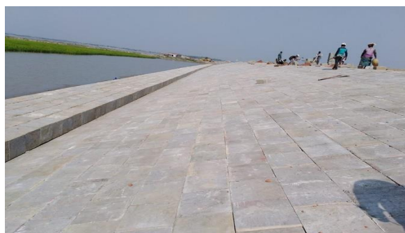
Figure 3-10: Completed Slope Protection Works in Polder-32
