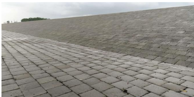
Figure 3-13: Nalian Closure Dam of Polder-32
