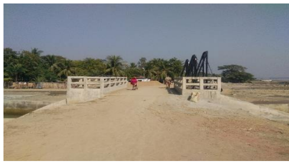
Figure 3-14: Completed DS-10 of Polder-33
