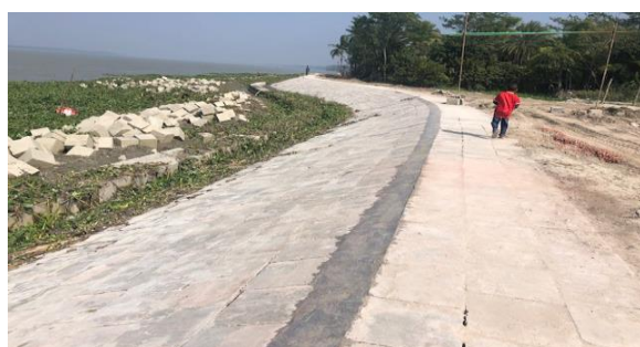
Figure 3-26: Bank Protection with Pitching Works (Polder 39/2C)
