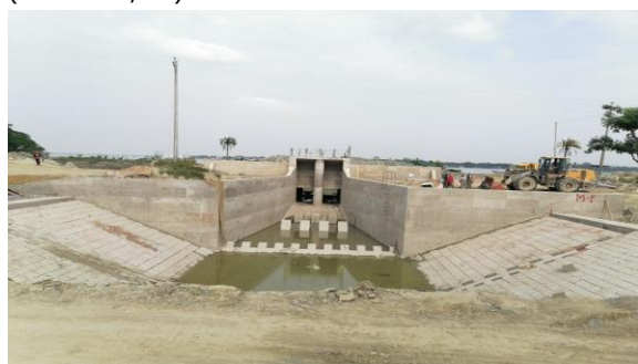
Figure 3-28: Ongoing DS-3 In Polder-43/2C
