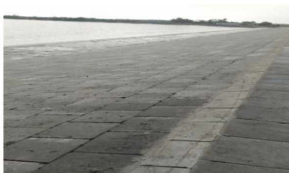
Figure 3-12: Nalian Closure Dam of Polder-32 (completed)
