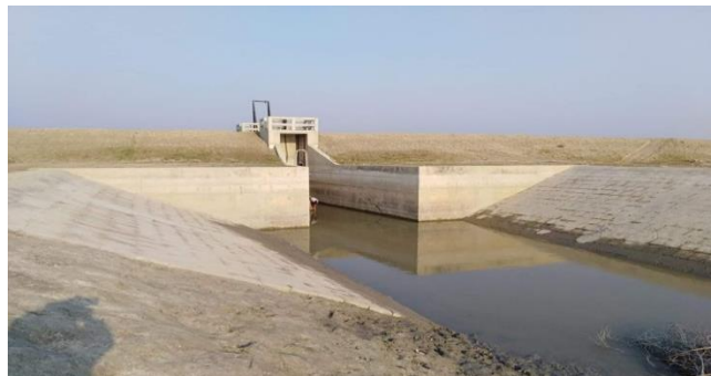
Figure 3-9: Completed DS of Polder-32
