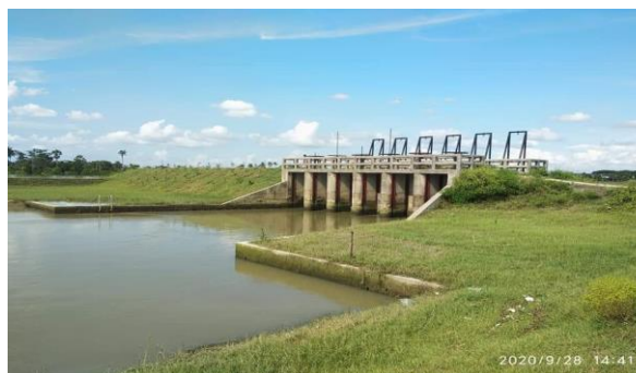
Figure 3-16: DS-6 of Polder-35/3 (Completed)
