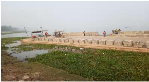
Figure 3-30: Dumping the cc block work at km 53+390-53+418 in Polder 39/2C
