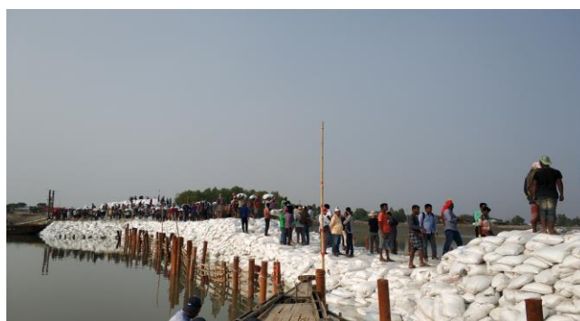
Figure 3-11: Nalian Closure Dam of Polder-32 (completed)
