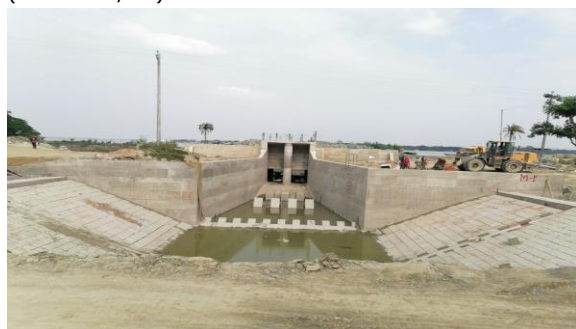
Figure 3-28: Ongoing DS-3 In Polder-43/2C
