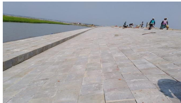
Figure 3-10: Completed Slope Protection Works in Polder-32
