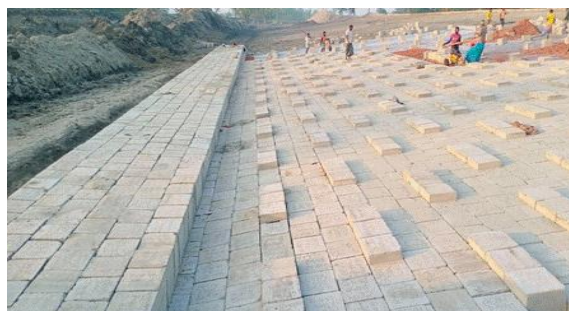
Figure 3-27: Ongoing Slope Protection Works (Polder 40/2), Barguna
