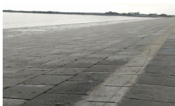
Figure 3-12: Nalian Closure Dam of Polder-32 (completed)
