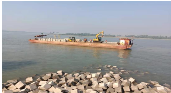
Figure 3-31: Dumping the cc block work at km6+150-6+710 in Polder-47/2
