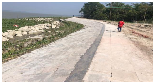
Figure 3-26: Bank Protection with Pitching Works (Polder 39/2C)
