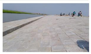
Figure 3-10: Completed Slope Protection Works in Polder-32
