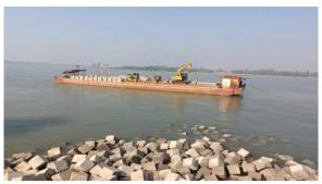
Figure 3-31: Dumping the cc block work at km6+150-6+710 in Polder-47/2
