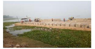
Figure 3-30: Dumping the CC block work at km 53+390 to km 53+418 in Polder 39/2C
