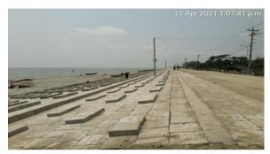
Figure 3-30: Slope Protection work For KM 30+800 to Km 31+450 in Polder-48
