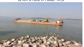
Figure 3-31: Dumping the CC block work at km6+150 to km 6+710 in Polder-47/2
