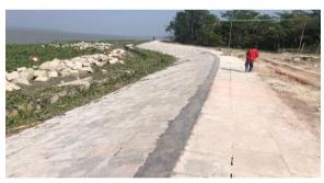
Figure 3-26: Bank Protection with Pitching Works (Polder 39/2C)
