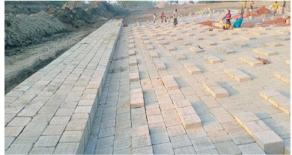
Figure 3-27: Ongoing Slope Protection Works (Polder 40/2), Barguna
