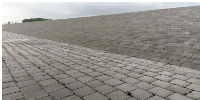
Figure 3-13: Nalian Closure Dam of Polder-32
