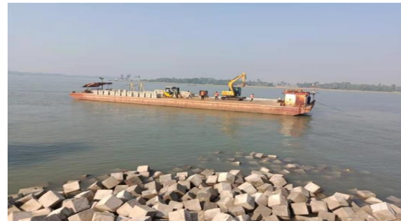
Figure 3-31: Dumping the CC block work at km6+150 to km 6+710 in Polder-47/2
