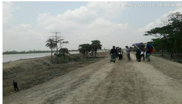
Figure 3-29: Retired embankment from Km 6+150 to Km 6+830 in Polder-47/2
