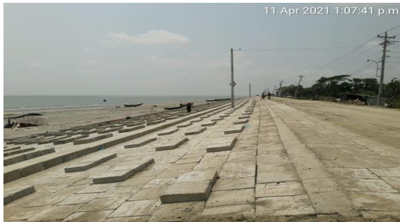
Figure 3-30: Slope Protection work For KM 30+800 to Km 31+450 in Polder-48
