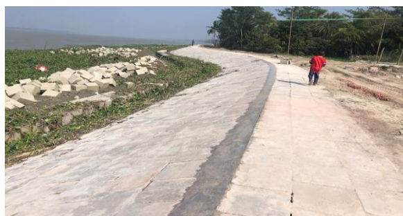
Figure 3-26: Bank Protection with Pitching Works (Polder 39/2C)
