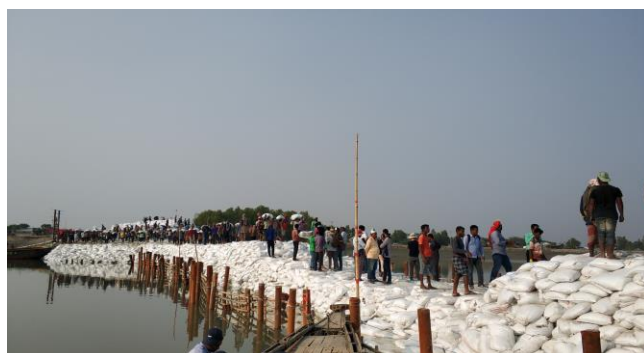
Figure 3-11: Nalian Closure Dam of Polder-32 (completed)
