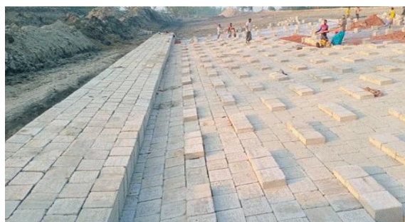
Figure 3-27: Ongoing Slope Protection Works (Polder 40/2), Barguna
