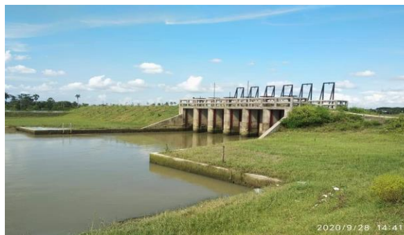
Figure 3-16: DS-6 of Polder-35/3 (Completed)
