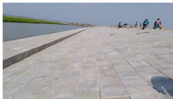
Figure 3-10: Completed Slope Protection Works in Polder-32
