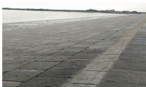
Figure 3-12: Nalian Closure Dam of Polder-32 (completed)
