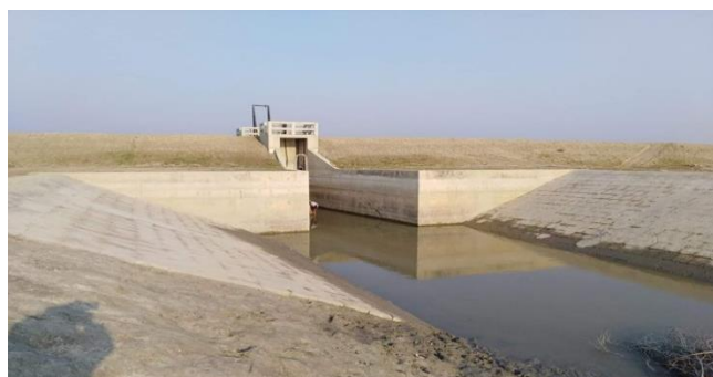
Figure 3-9: Completed DS of Polder-32
